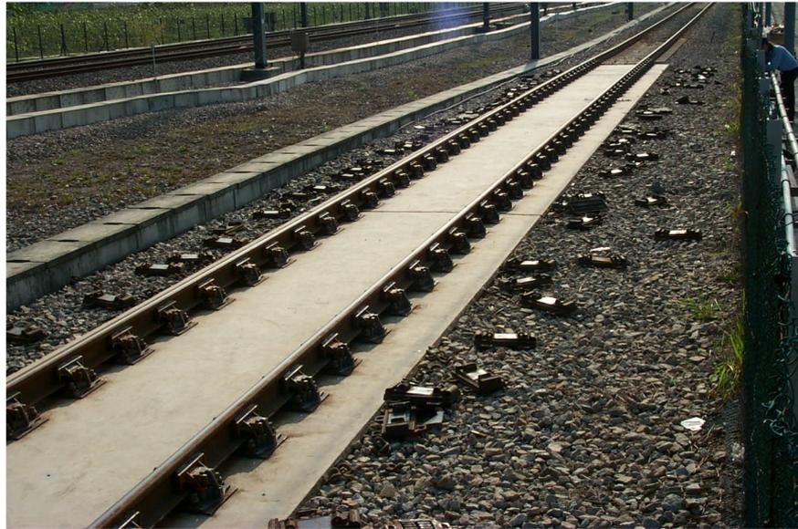
Figure 1.4. An example of a directly fastened track form in Hong Kong.
