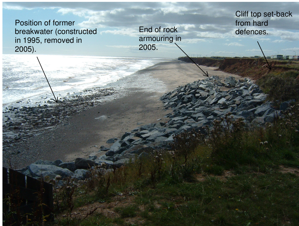
Figure 4.37 – The rock armour extensions at Withernsea and subsequent shoreline set-back. Photograph taken 9 th August 2006.
