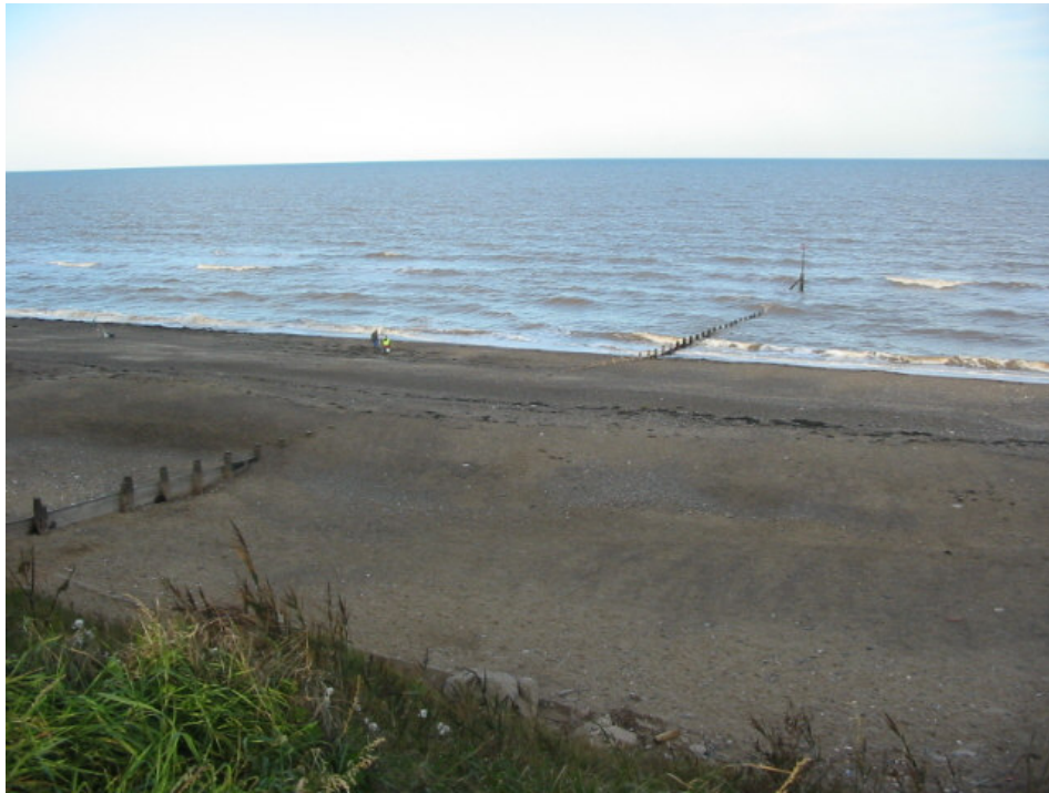
Figure 4.24 – Hornsea's up-drift groyne. Sediment has accumulated up-drift of the defences, creating a wide, high beach protecting the cliffs from marine attack. (Photograph taken by Max Barton on 1 st October 2007).
