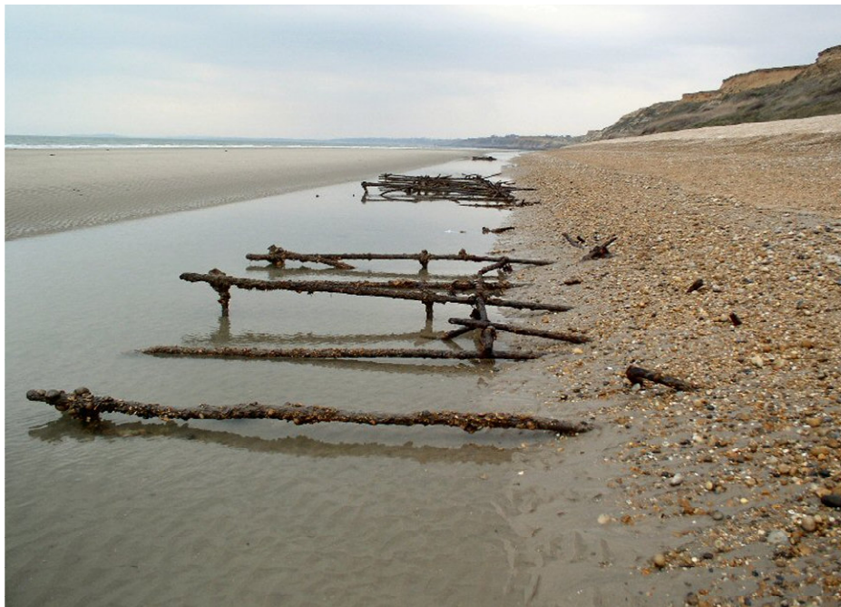
Figure 6.14 – Abandoned World War 2 scaffolding at Milford-on-Sea, Christchurch Bay. Now located in water between the beach and the offshore bar, it raises the issue of safety of abandoned defences. Photograph taken 10 th March 2005 by Ian West (West, 2008).
