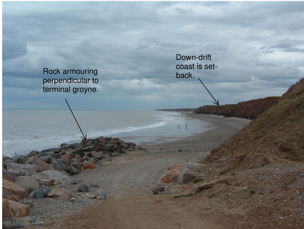
Figure 4.27 – Cliff set-back down-drift of Mappleton. Photograph taken 10 th August 2006.
