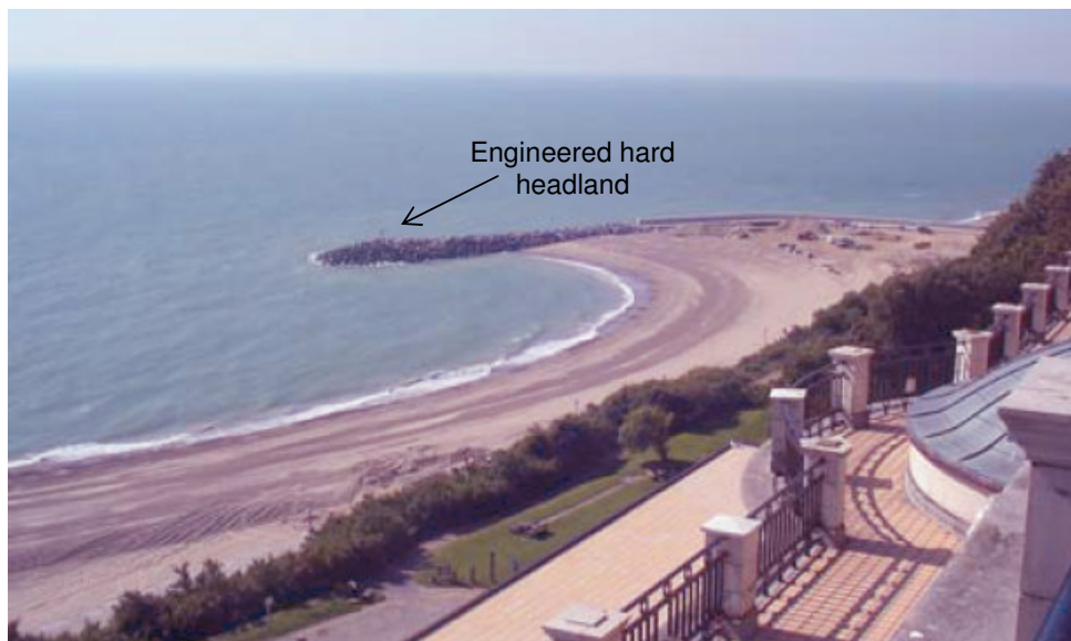
Figure 2.19 – An artificially stable crenulate shaped bay south-west of Folkestone, Kent. Once the headlands were created the beach was nourished. Sediment was designed to be contained within the bay (known as static equilibrium), creating a wide beach protecting the seawall (Channel Coastal Observatory, 2005a).
