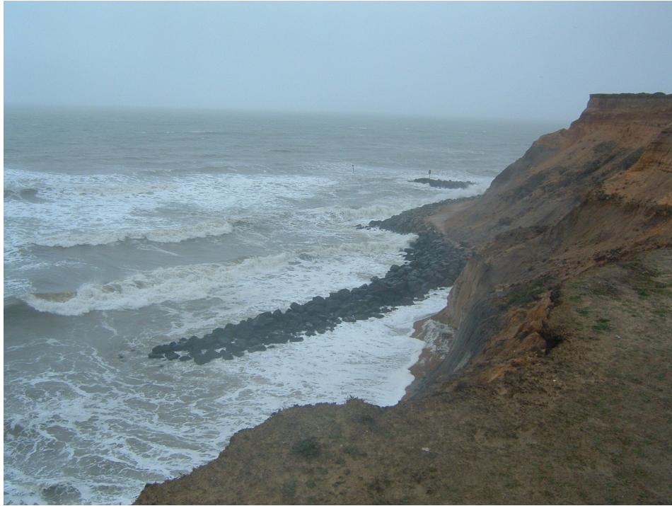
Figure 5.25 – Wave attack on the cliff base behind the rock armouring at Barton-on-Sea. The armouring was originally placed against the cliff base to protect it from erosion. The cliff continued to erode and in 2005 there was a distance of 22m between the cliff base and the armouring as it became outflanked. Photograph taken 31 st March 2006.
