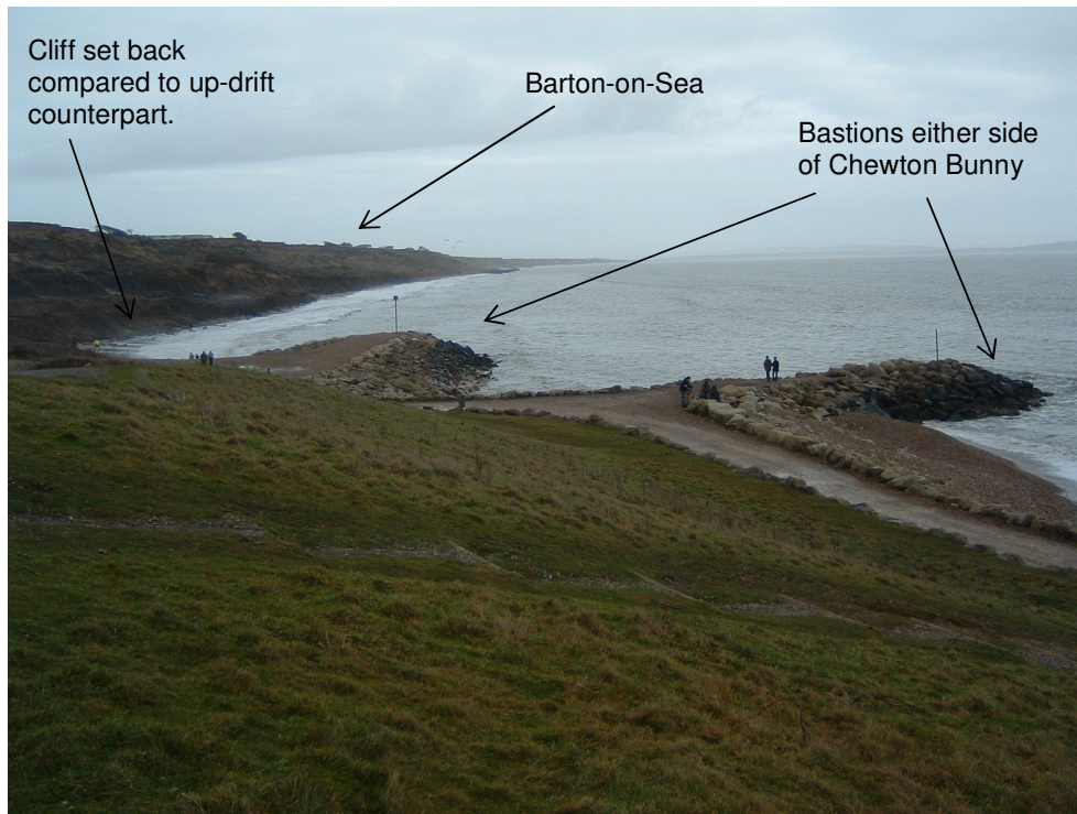
Figure 5.15 – Down-drift of the Highcliffe defences. The Chewton Bunny bastion acts as the terminal groyne with the cliff set back down-drift. Longshore drift is eastwards, into the photograph (photograph taken 26 th December 2007).
