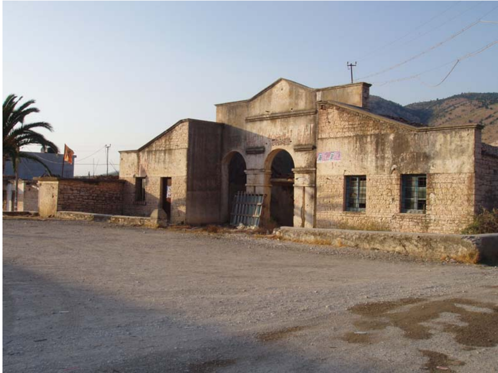
Figure 7.29 The central square of the village of Mursia.
