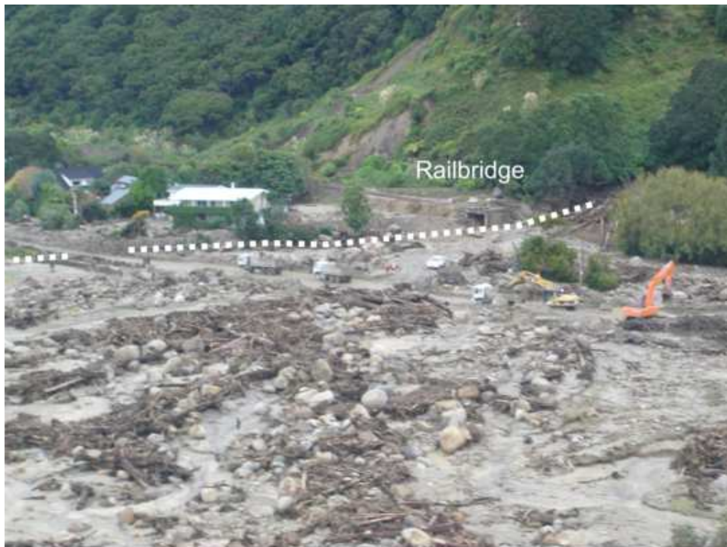
Fig. 4. Aerial Photograph (courtesy Terrain Consultants) showing in detail where the debris flow emerged from the confinement of the Awatarariki Stream. The first debris-laden currents passed beneath the railroad bridge and followed an existing stream channel (white dotted line). After debris build-up behind the bridge and its failure, the main debris flow bypassed the channel and spread out in an unconfined way across the pre-existing fan with large truck-sized boulders visible in the proximal fan. Remediation efforts had just commenced when this photograph was taken.
