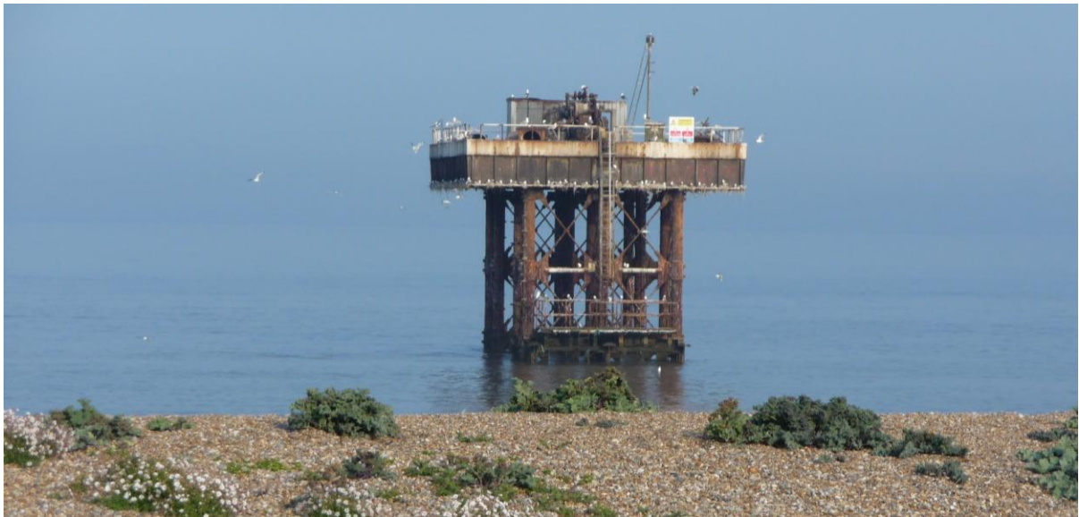
Plate 2 Structure surrounding the Sizewell B cooling water intake
