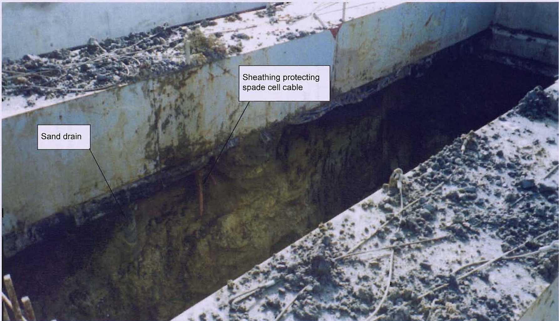
Figure 3-31: Photo showing sand drain and cable for spade cell 11 (taken on 13 th February 2001 – Day 495)
