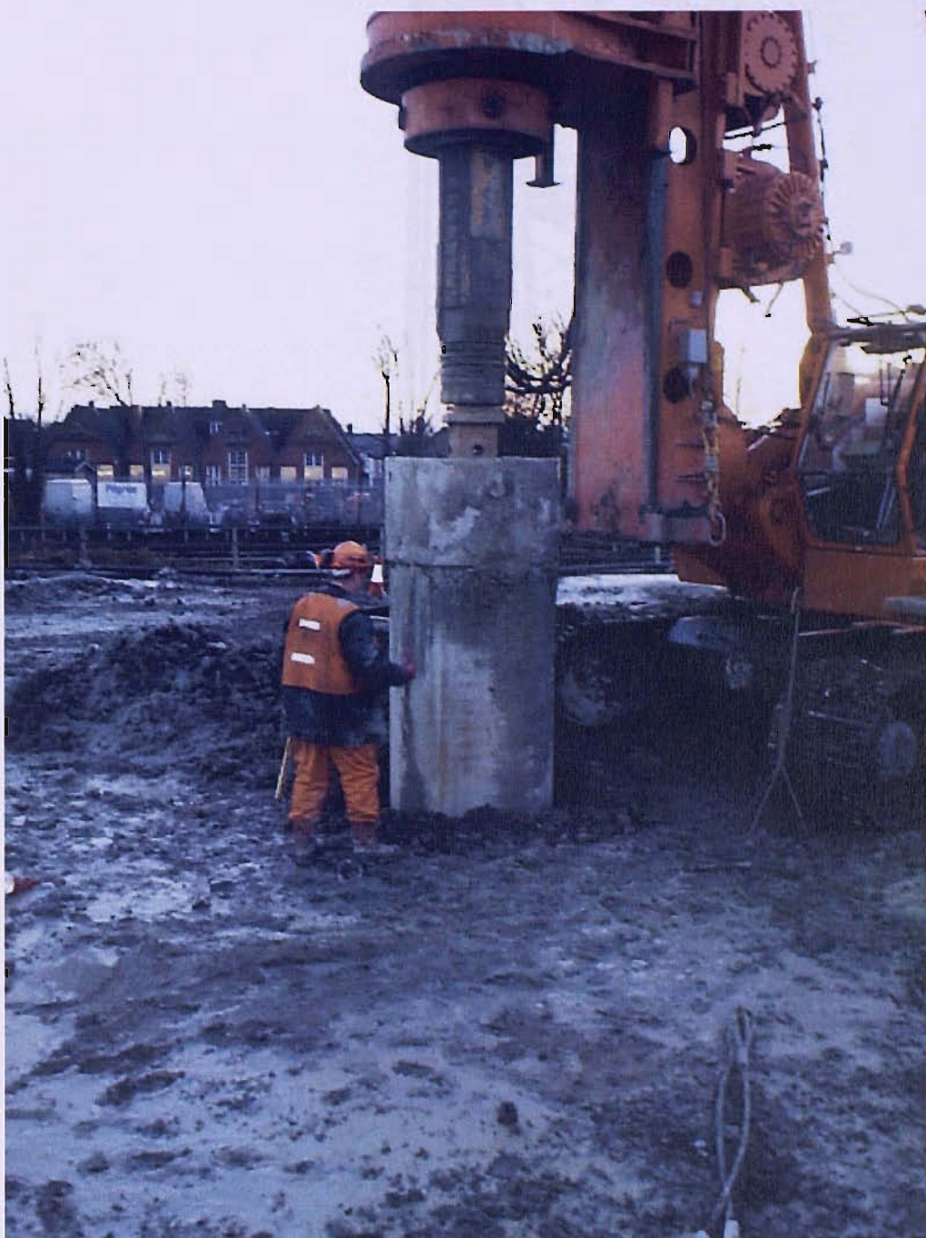
Figure 3-27: Installation of casing
