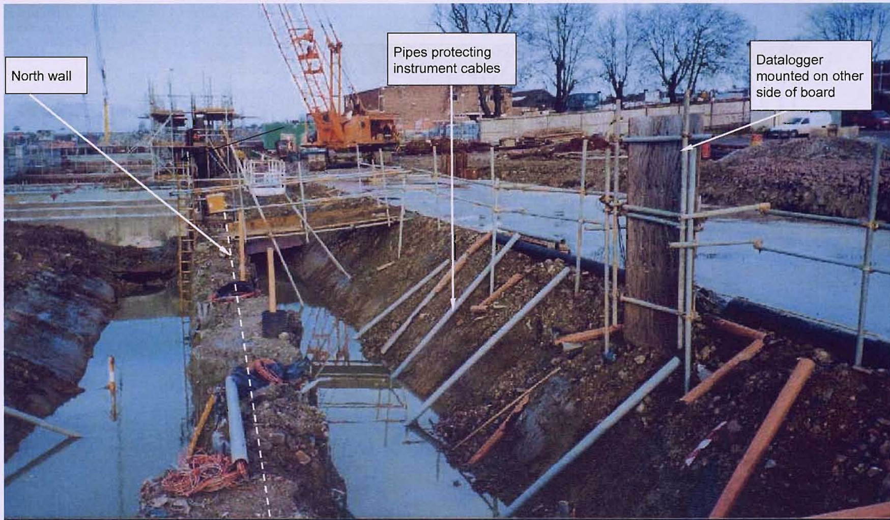
Figure 3-33: Excavation either side of the north wall before break down to level of capping beam (taken on 1 st November 2000 – Day 391)
