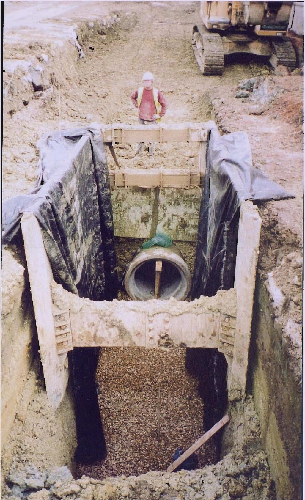
Figure 3-48: Storm drain installed behind north wall in November 2001 (Day 864)
