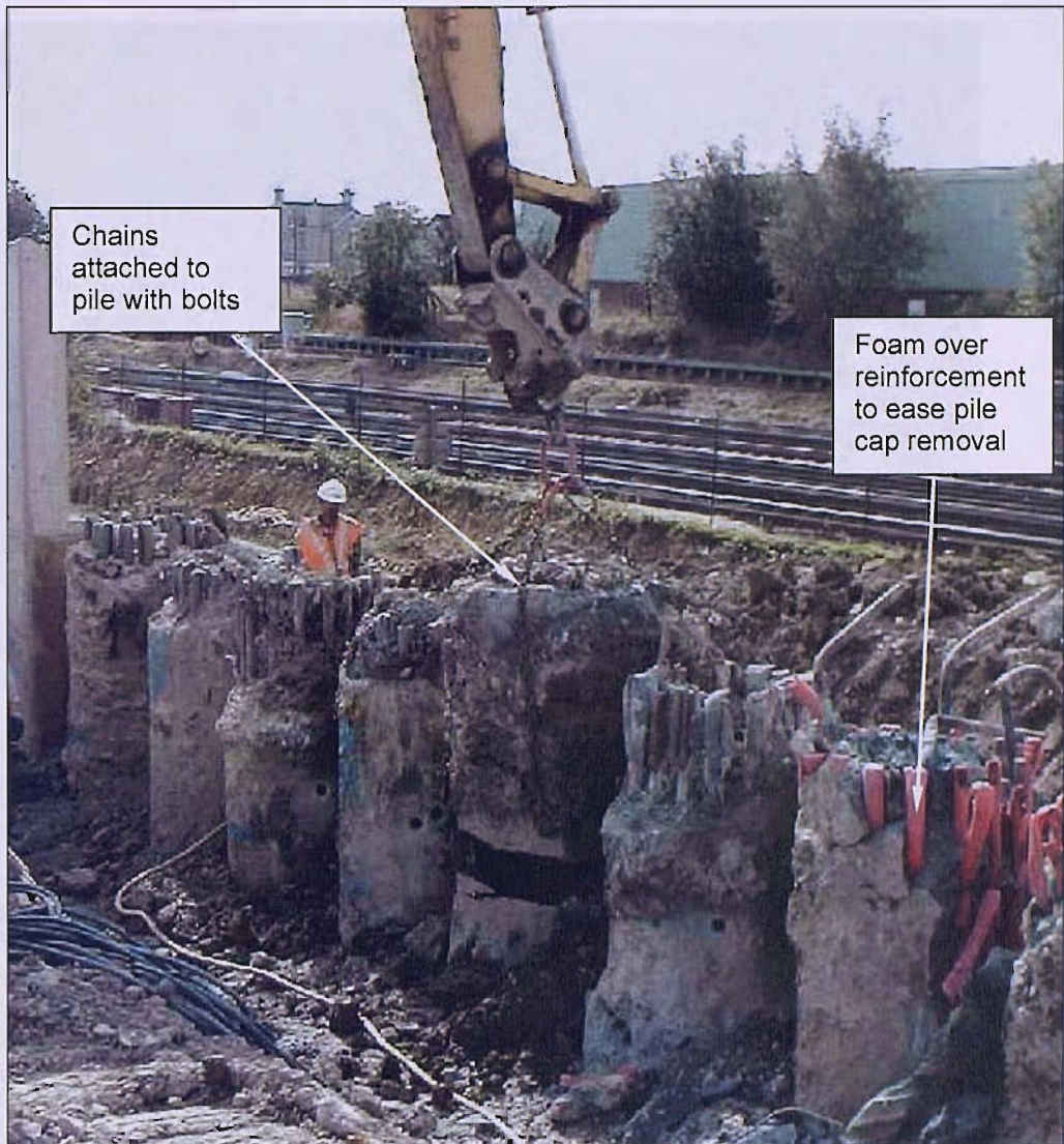
Figure 3-34: Pile top removal (south wall) (taken on 31 st August 2000 – Day 329)
