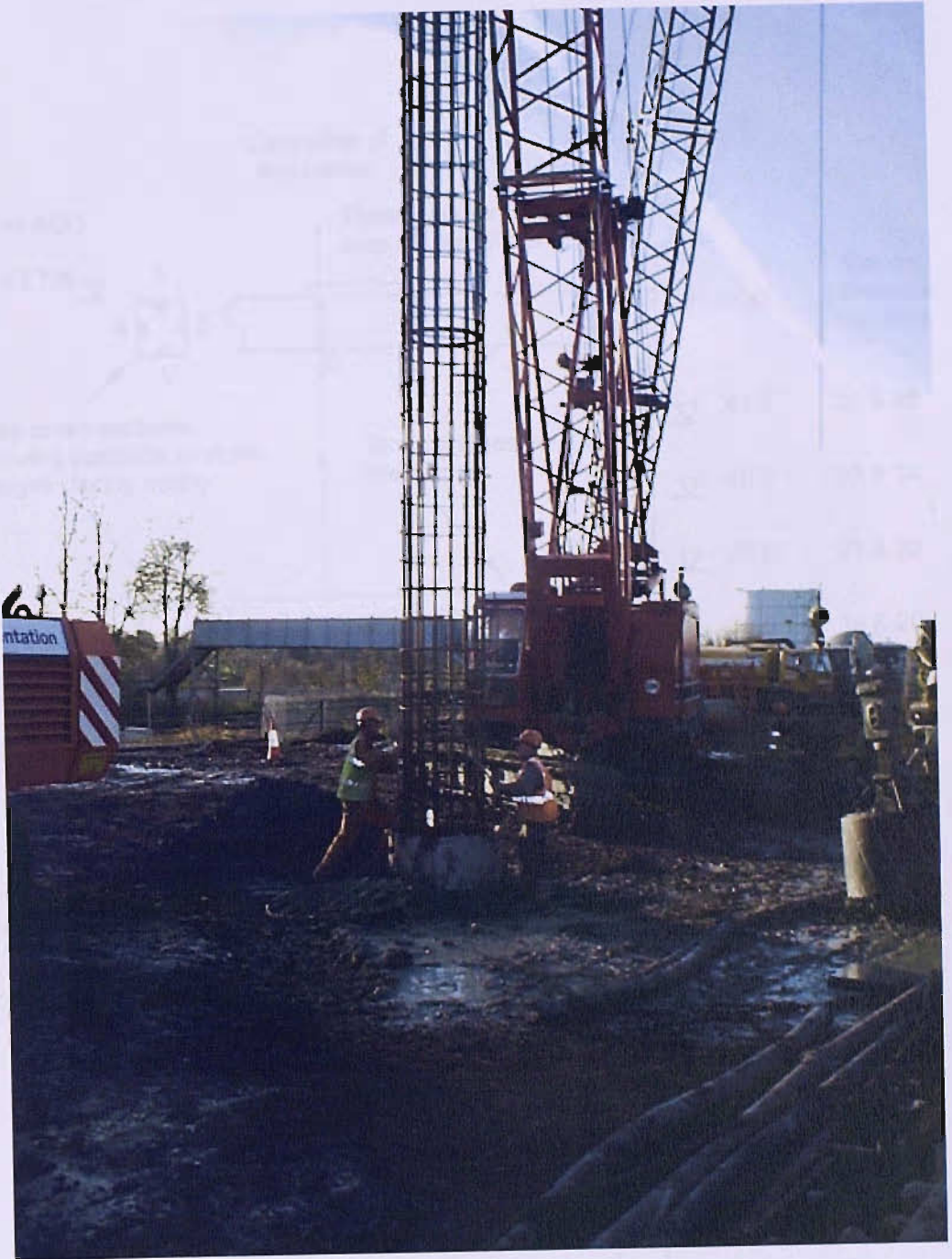
Figure 3-28: Installation of reinforcement cage
