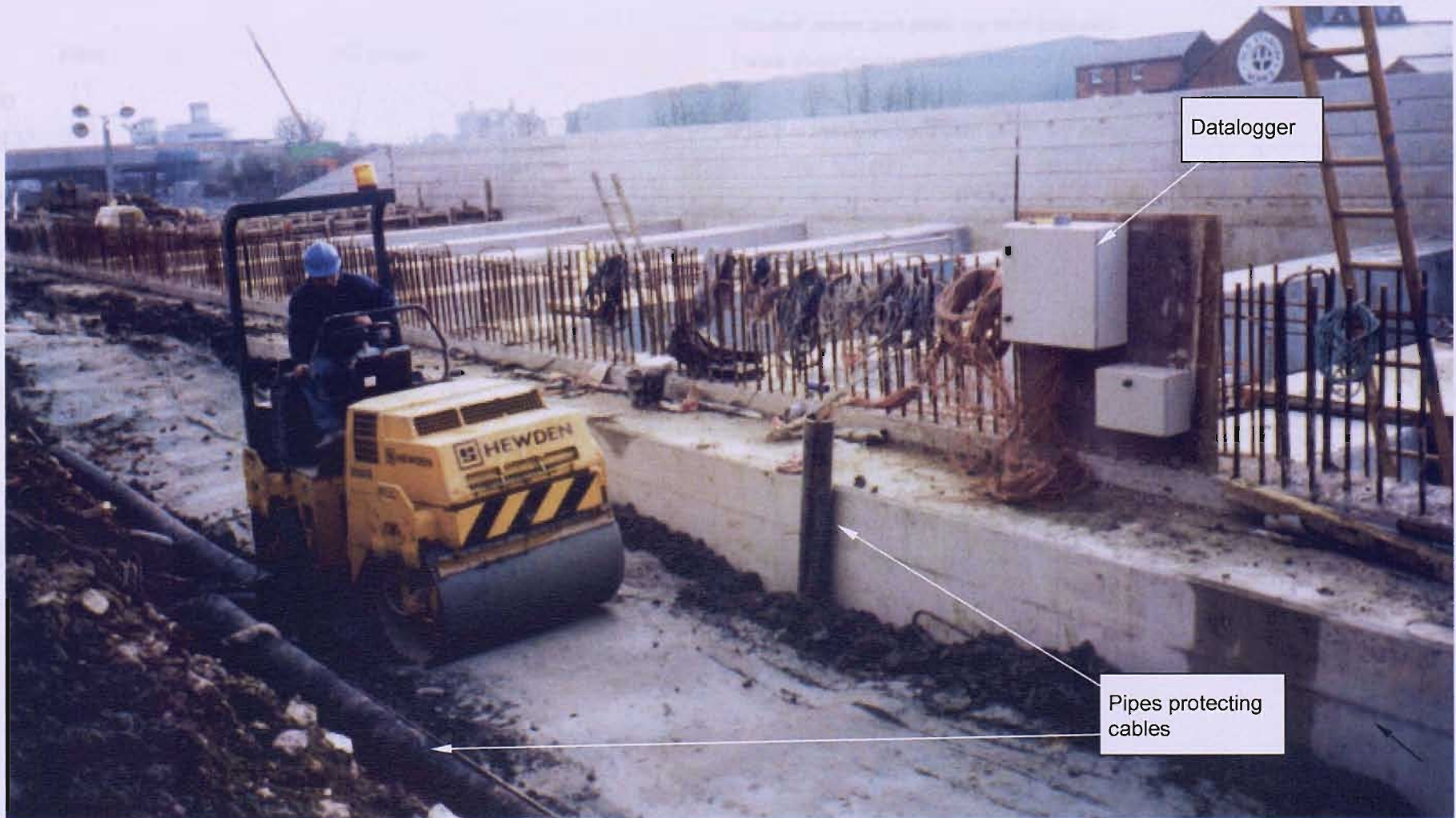
Figure 3-41: Compacting backfill in the instrumented section (taken on 29 th January 2001 – Day 480)
