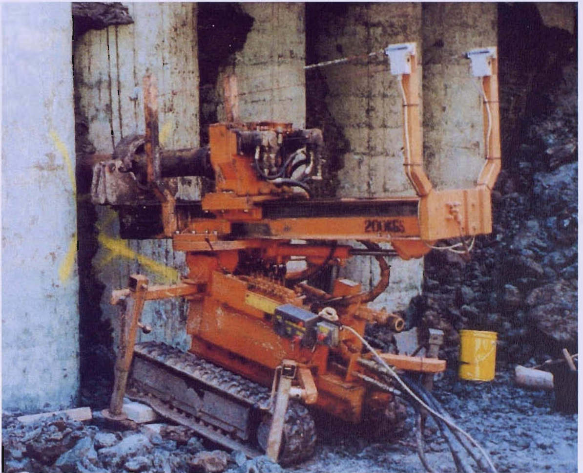
Figure 5-3: Equipment for drilling horizontal borehole
