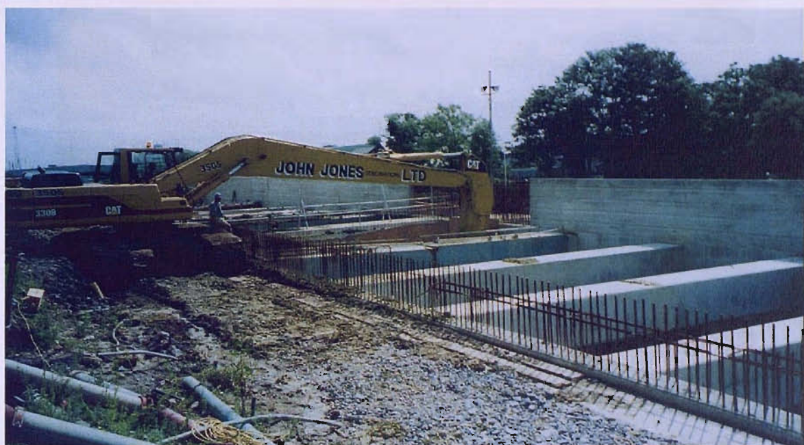
Figure 3-43: Excavation using long-reach excavator
