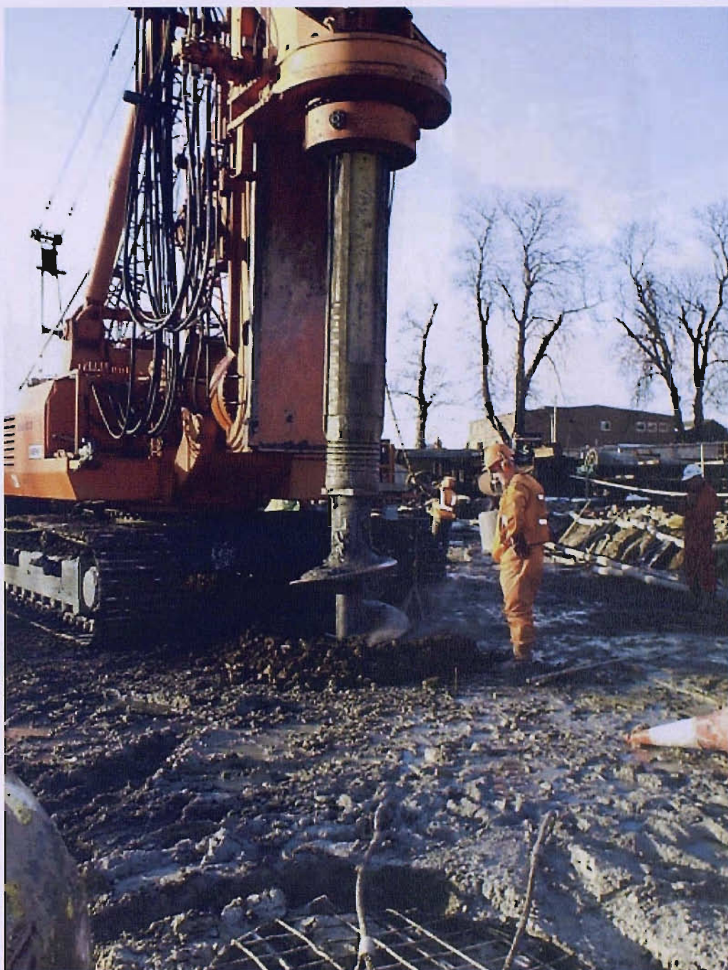
Figure 3-26: Pile boring
