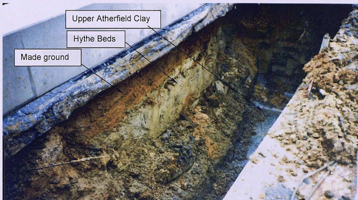
Figure 3-7: Looking into the cutting between RC props during excavation
