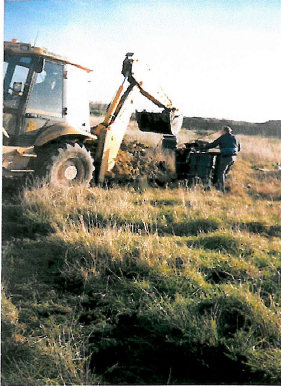
Plate 5.2a: Loading of spoil into the drums
