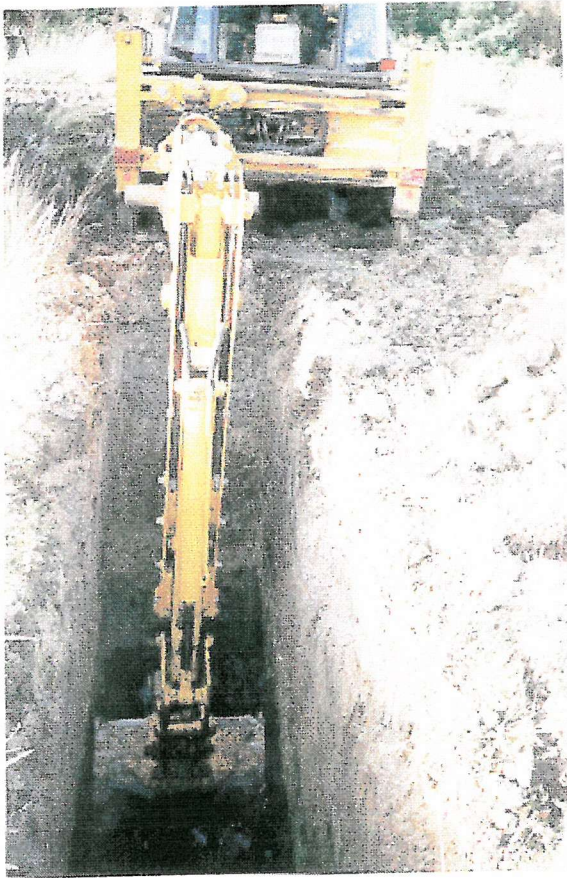
Plate 5.1a: Excavation of a uniform void.
