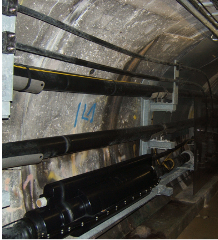
FIGURE 1.2: 400kV XLPE cable installation in a tunnel
