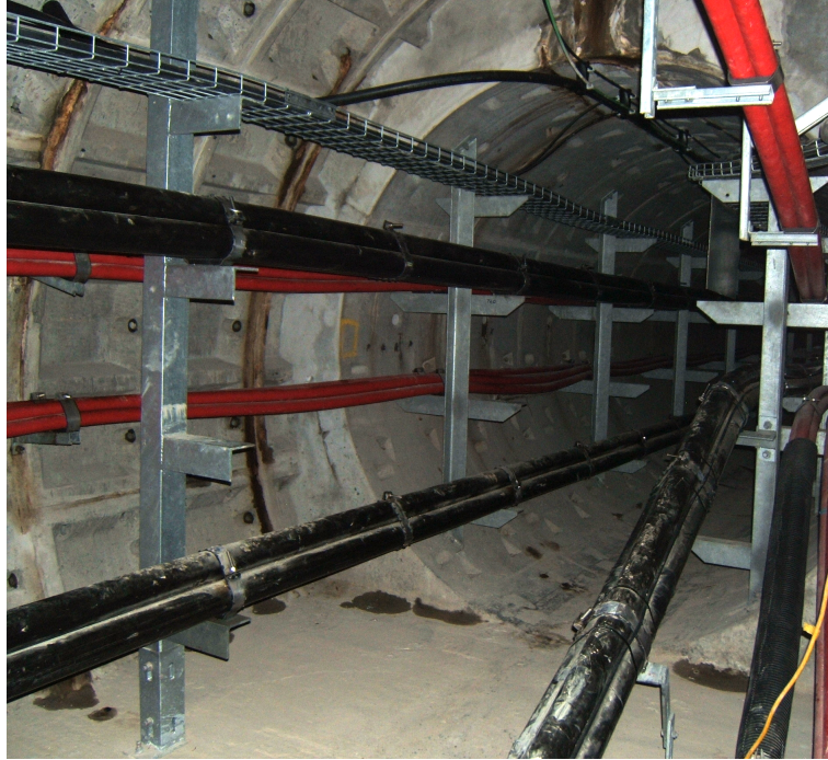
FIGURE 2.2: Cable tunnel with co-located 11kV and 132kV circuits
