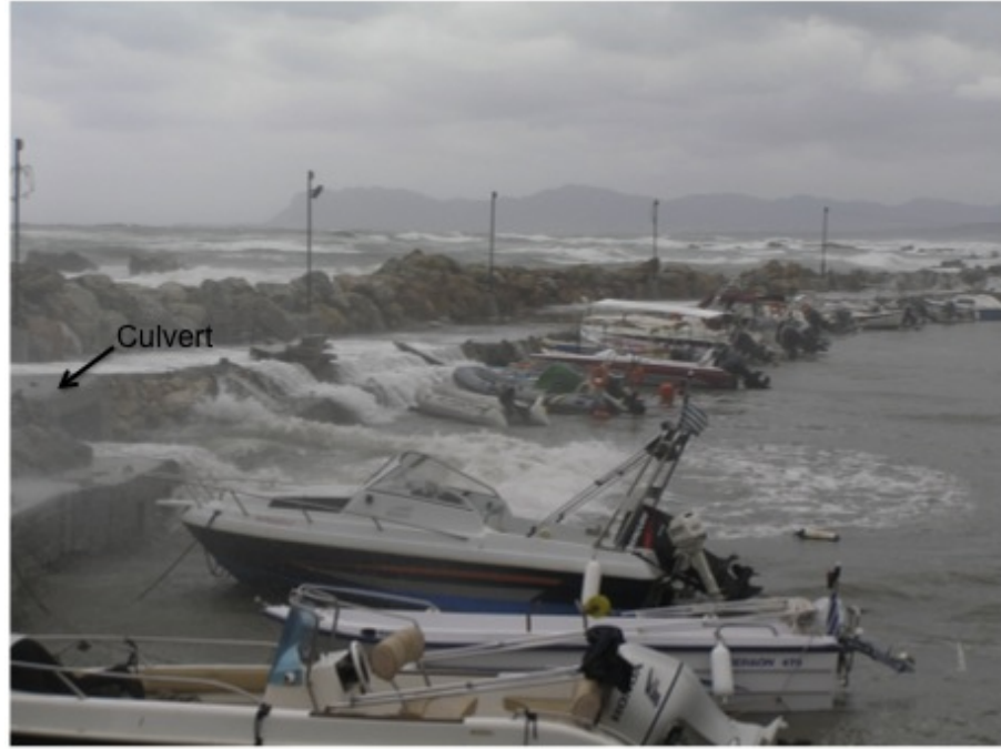
Figure 6.1: Photograph of a wave passing through a culvert placed at MWL during a storm event, North Crete, Greece
