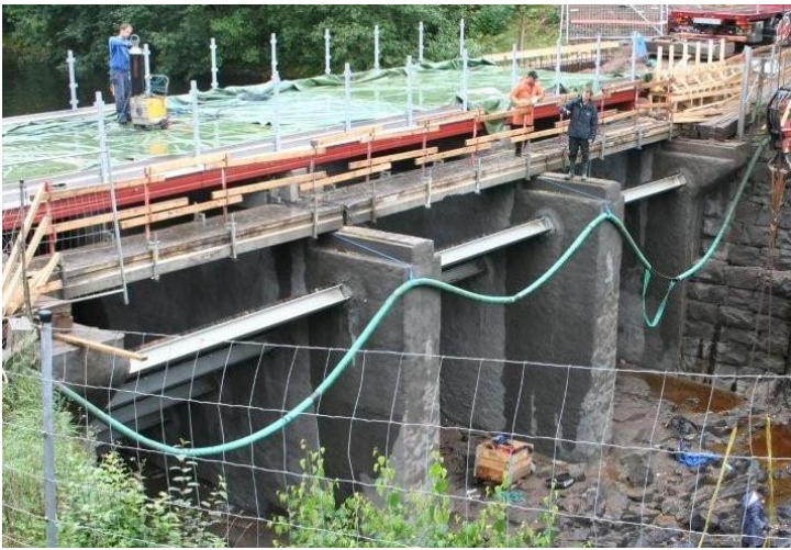
Plate 1.3 Replacement screens installed at the Ätrafors power plant on the River Ätran, Sweden during 2008 to improve safe passage of European eel, Anguilla anguilla (photos courtesy of Olle Calles, taken 2008).
