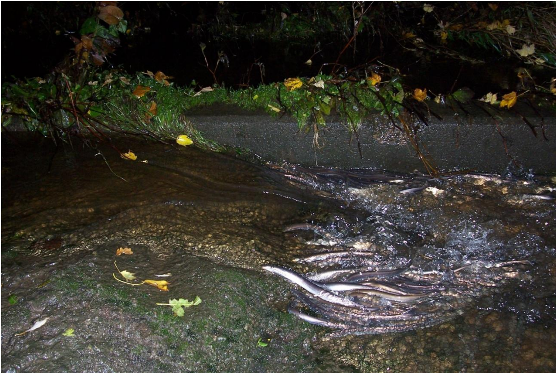
Plate 1.1. Fish pass at Acaster Malbis on the Yorkshire River Ouse. A large number of river lampreys, Lampetra fluviatilis , are accumulated downstream (photo taken November 2008).
