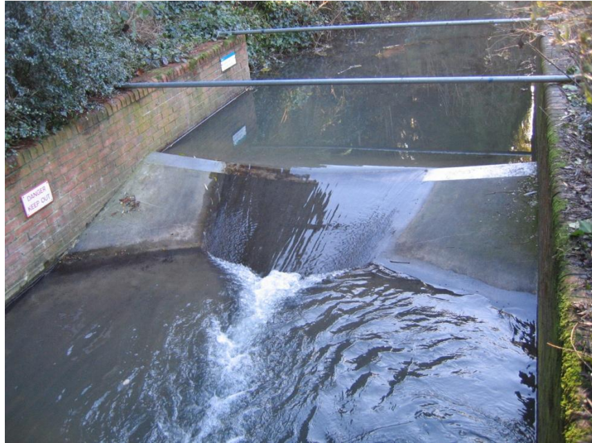
Plate 9.1 Flat-v weir under low discharge conditions at Kingsclere, UK (photo taken January 2008).
