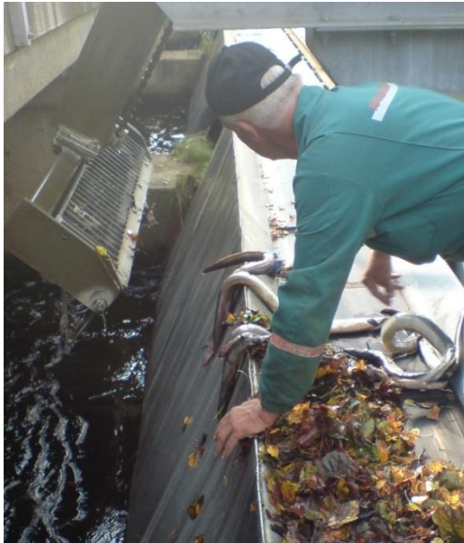
Plate 1.2 European eel, Anguilla anguilla , mortalities due to impingement at the Ätrafors power plant screen on the River Ätran, Sweden, prior to replacing the screen in 2008 (photos courtesy of Simon Karlsson, taken 2007).
