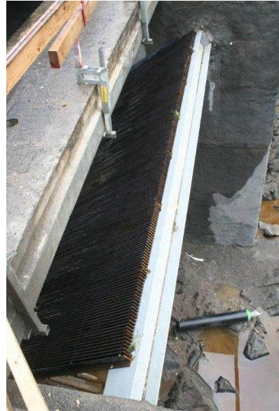
Plate 1.3 Replacement screens installed at the Ätrafors power plant on the River Ätran, Sweden during 2008 to improve safe passage of European eel, Anguilla anguilla (photos courtesy of Olle Calles, taken 2008).
