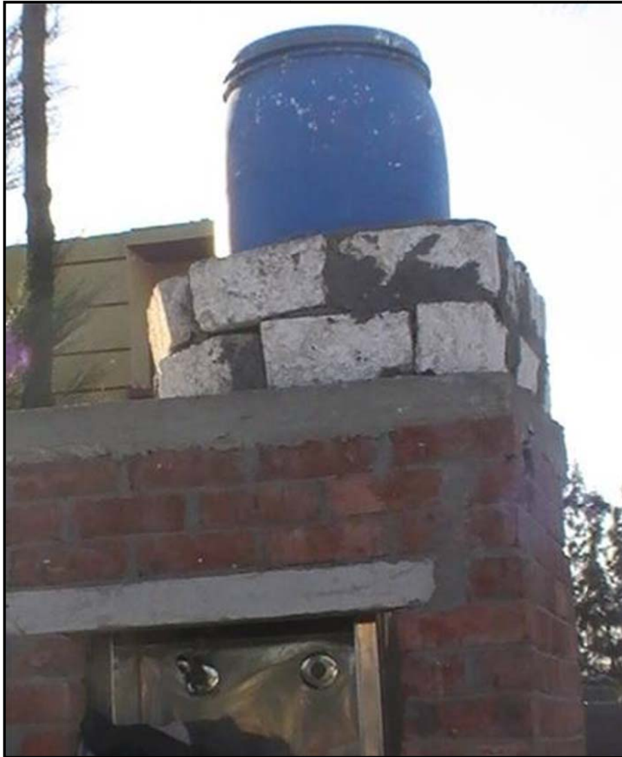
Figure 3.13 Picture shows a form of public drinking water provision, the electrical cooler (Coldair) which is used instead of the more traditional Zir vessel
