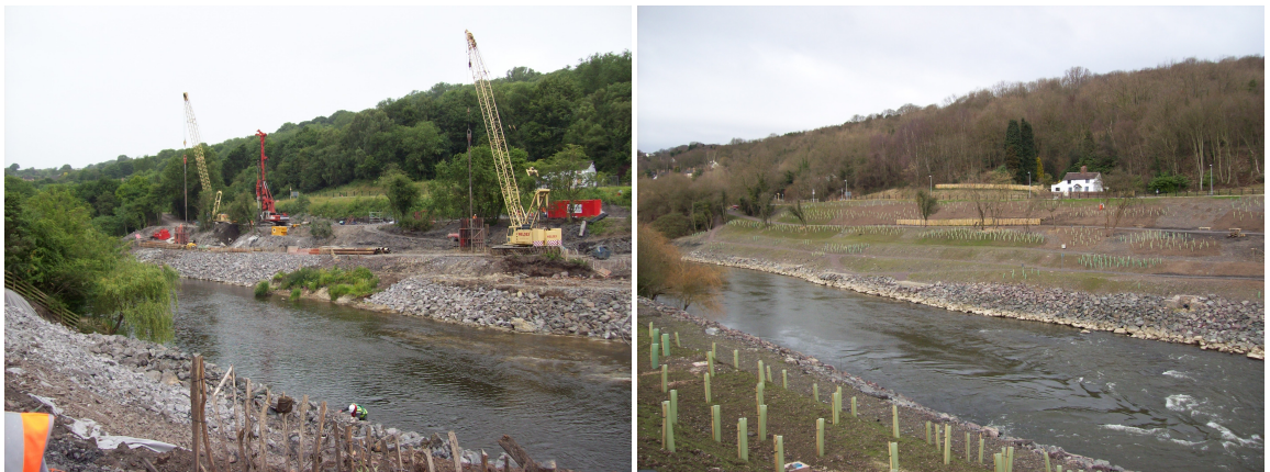
Figure 1.1: Ironbridge stabilisation works, during the installation of the piles (left) and after the completion (right).
