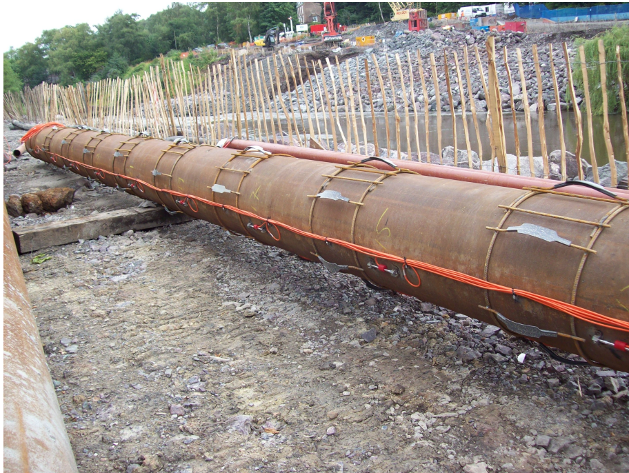
Figure 5.12: Ironbridge instrumented pile. Spacers are welded to the steel reinforcement pipe to keep it in position during installation. They also act as bonding points for the external grout ring.
