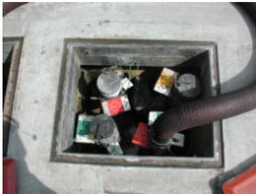
Plate 2. Manhole and offset fill pipes. Those not in use have caps in place. Ignition incident occurred with No. 2 (bottom left).
