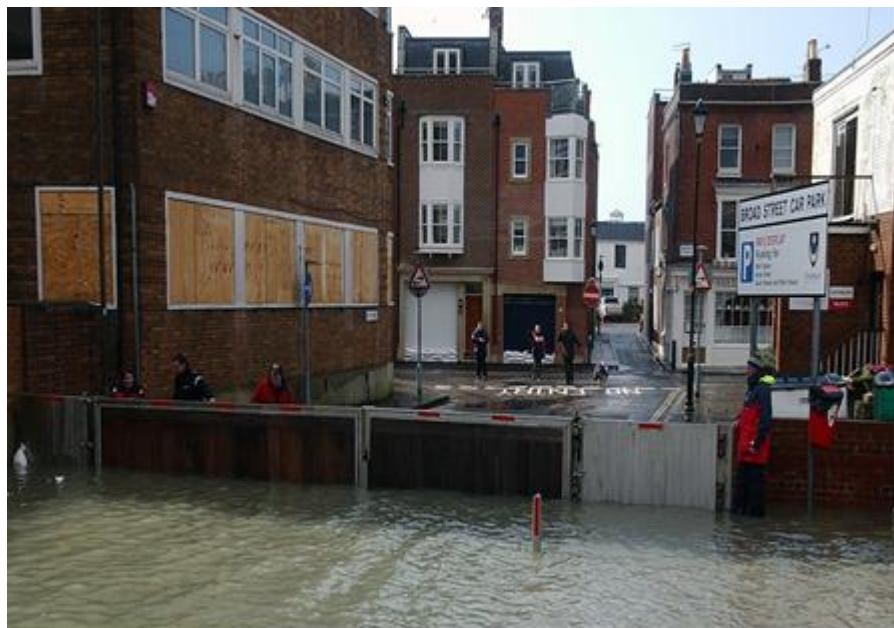
Figure 7-5 A flood barrier deployed in Portsmouth (photograph courtesy CDP)
