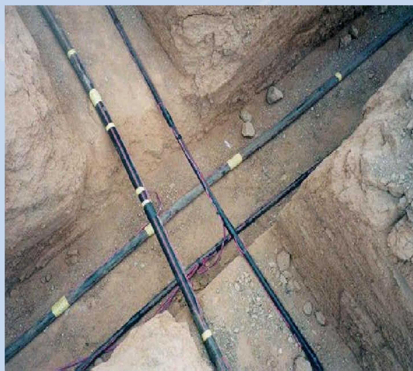
Figure 1 - sample cable crossing in North America (www.dstar.org/research/project-desc/UG-cable-ampacity)
