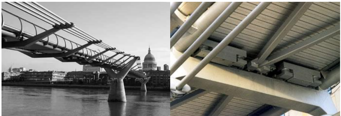
Figure 7.3: Millennium Bridge London (right picture) with DVA mounted beneath the deck to reduce its vibration level (left picture) from [59].
