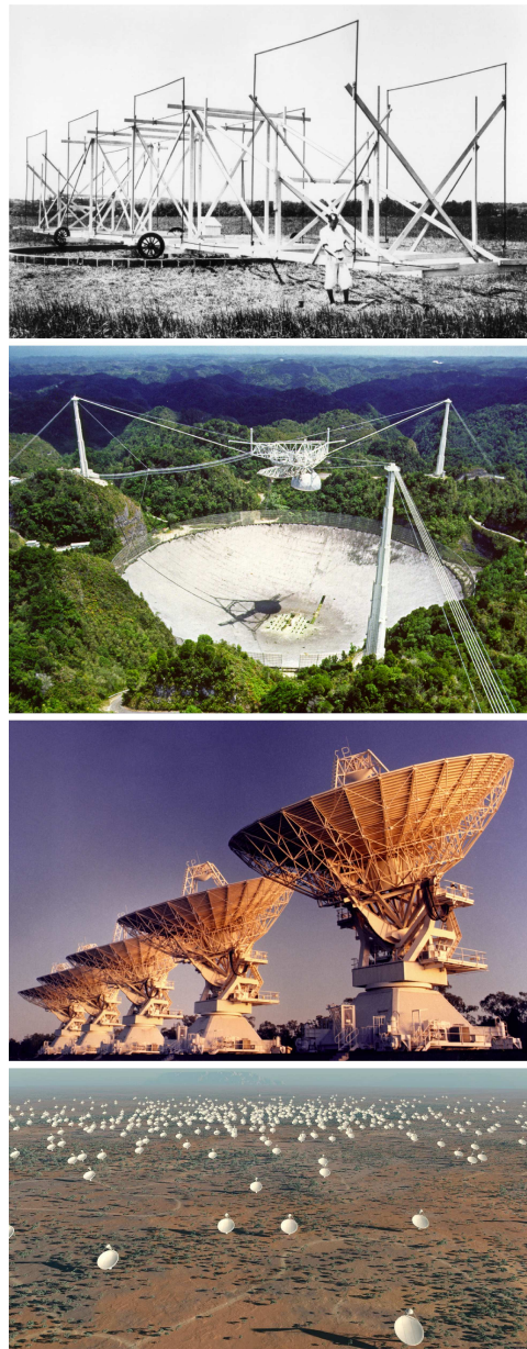
Figure 1.1: Radio telescopes of the past, present and future. From the top down, first panel: Jansky's 'merry-go-round', a turntable mounted antenna with a diameter of approximately 30m that was originally located at Bell Telephone Laboratories in New Jersey, USA. Second panel: The Arecibo Observatory, the largest single filled focusing dish on Earth with a diameter of 305m situated near Arecibo city, Puerto Rico. Third panel: The Australia Telescope Compact Array (ATCA) which is made up of six 25m dishes (the sixth is fixed several kilometres from the five shown) which can have a maximum baseline of 6km, located in Narrabri, Australia. Final panel: An artist's depiction of the Square Kilometre Array (SKA) which could be made of thousands of small parabolic dishes spread over thousands of kilometres (the name itself refers to the array's proposed collecting area) to be split between Australia, New Zealand and South Africa.
