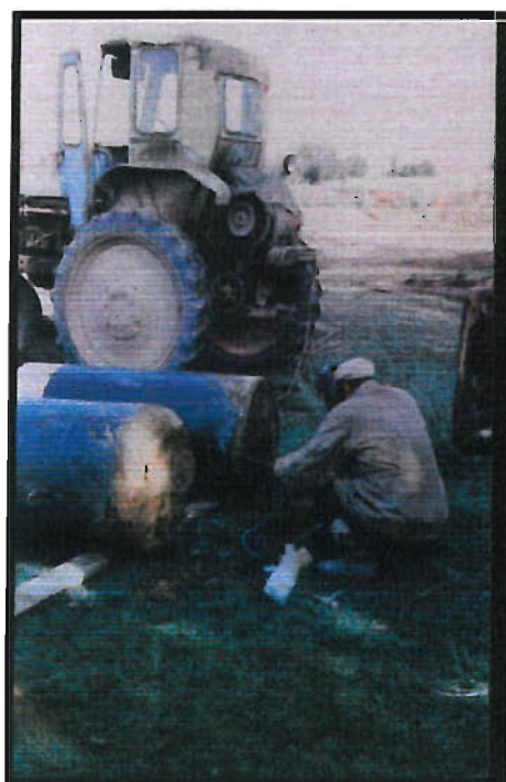
Plate A. Perforated Drainage Plate Welded to Bottom of Lysimeters
