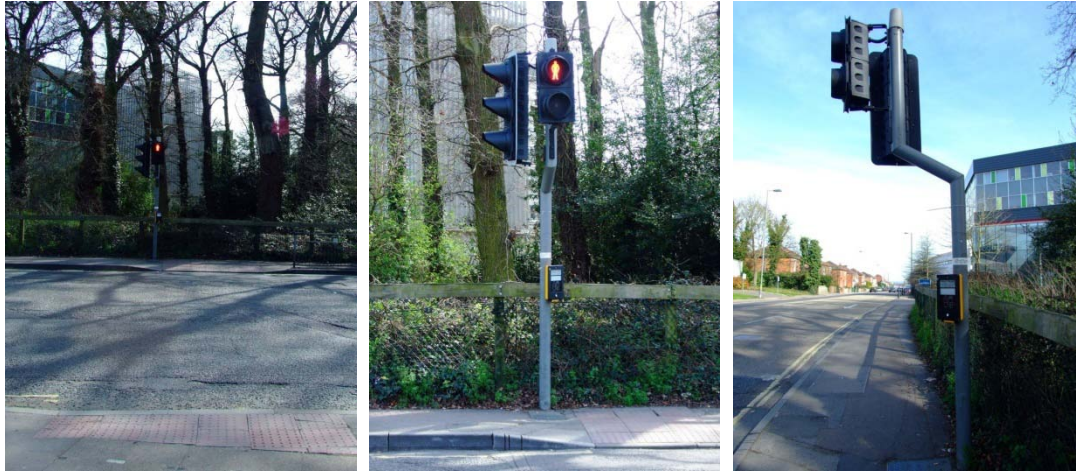
Figure 2.3 A typical Pelican crossing (Southampton, UK)
