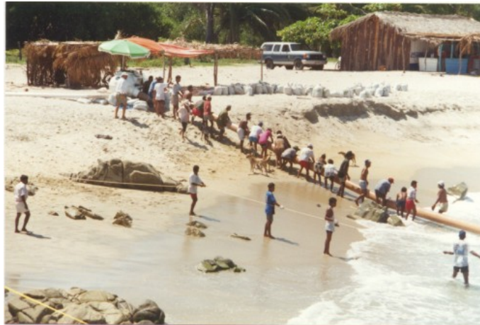
Figure 3.12: Installation of the SIBEO on the shore of Ensenada in Mexico. It can be seen how the device represents a simple low cost WEC of easy installation .(Czitrom et al., 2006)
