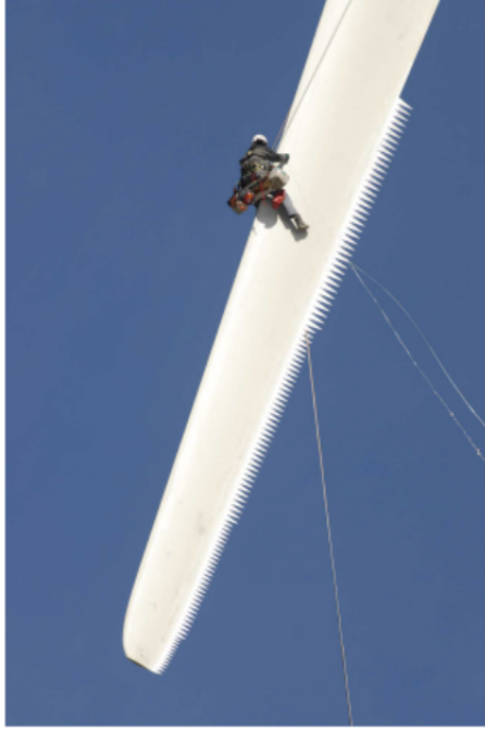
(a) Serrations on the full scale wind turbine.
