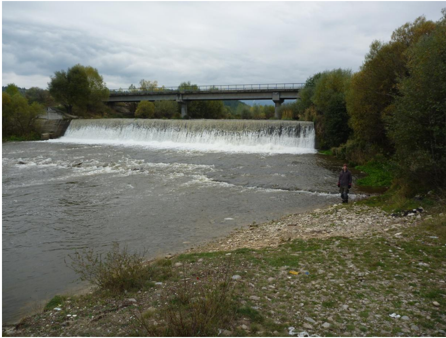
Figure 1.2 A broadcrest weir with a large height difference or ‘step’ between upstream and downstream water levels.
