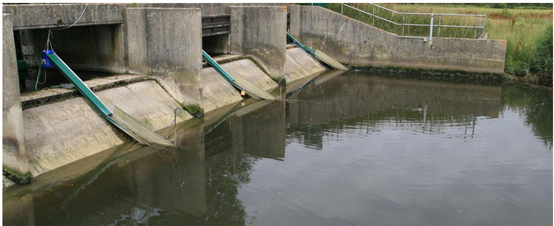
Figure 4.3 Eel traps located at Judas Gap intertidal weir, river Stour, Suffolk, UK.
