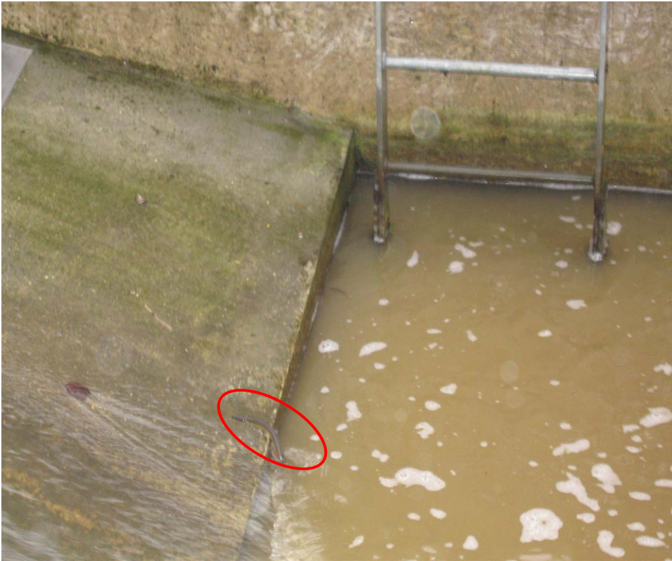
Figure 9.1 Eel attempting to ascend at the channel centre of a flat V triangular profile flow gauging weir, under summer low flow conditions.
