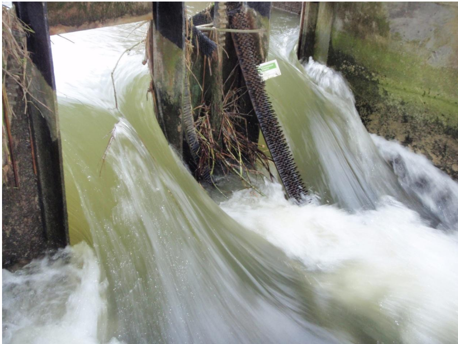
Figure 1.3 Flow constricted at an undershot sluice creates high water velocity downstream of the structure.
