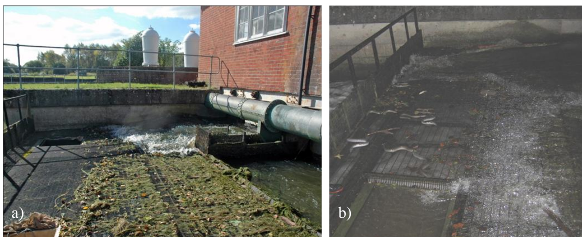
Figure 4.4 a) Eel rack with water spilling from undershot sluice gates (right-hand side) onto mesh deck with catch boxes, Longham, river Stour, Dorset, UK, b) Eels captured on the rack during night-time operation (photo courtesy of Roger Castle).
