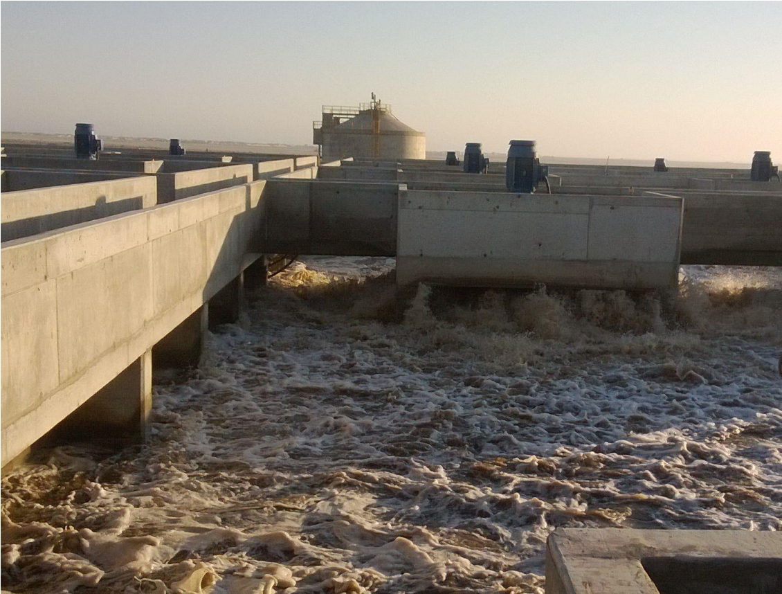
Figure 32 Aeration of wastewater at Swakopmund wastewater treatment plant
