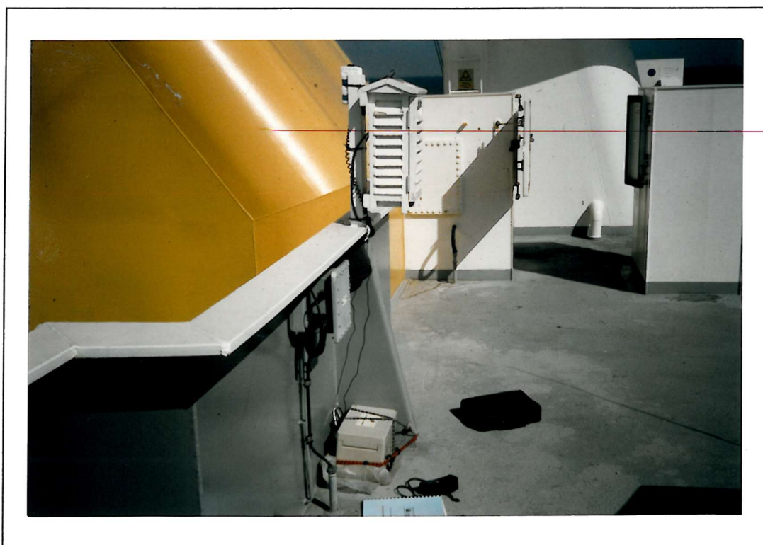
Figure 4.12 Installation of the TASCO THI-500 IR radiometer on the 'Monkey island' aboard the RRS James Clark Ross .
