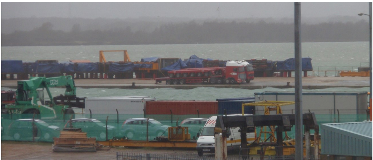
Figure 5.10 High water at Southampton docks (photo taken at 13:04, 10 March 2008 from the window of the Channel Coastal Observatory, National Oceanography Centre). The nearest peak still water level recording was 2.84 mODN (at Dock Head, ABP). The docks around this location are built to a level of approximately 3.3 to 3.6 mODN. This suggests a minimum freeboard of approximately 0.5 – 0.7 m, although the peaks of the oscillating water surface are seen to be level with the dock surface and sea water was observed to overtop onto the docks (although notable incidents of flooding were not reported here).
