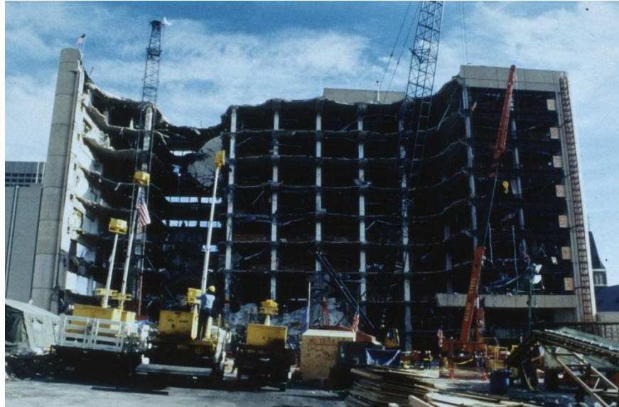
Figure 1-1: Extensive blast damage to the Murrah building, FEMA (1995)
