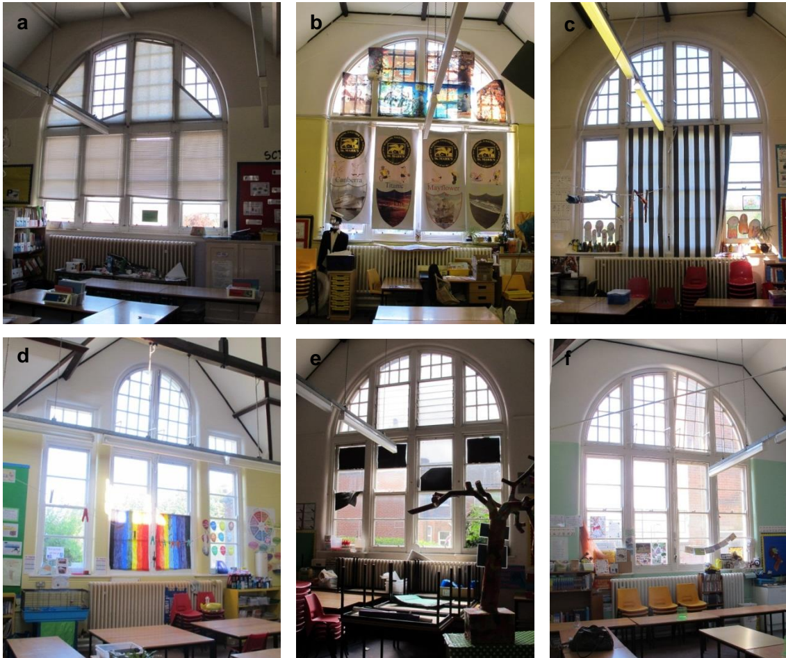
Figure 4.15. Window shading of 6 classrooms: a. shading blinds, b. canvas posters, c. fabric panels, d-e. carton boards, f. no shading.
