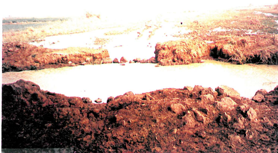
Plate10.3 Breach on the Lugu main canal due to cattle crossing
