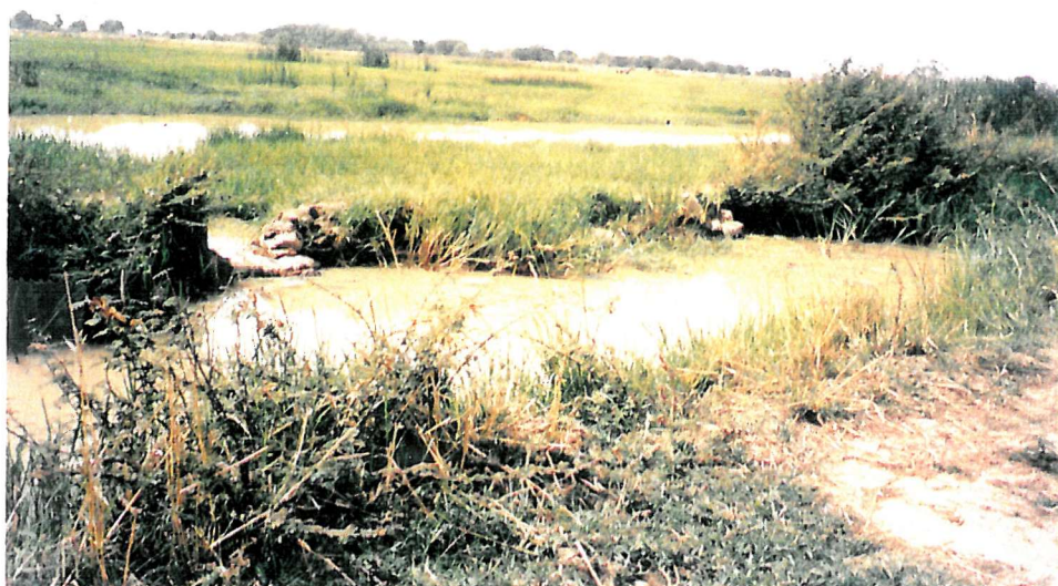
Plate10.4 Breach on the Tutudawa main canal
