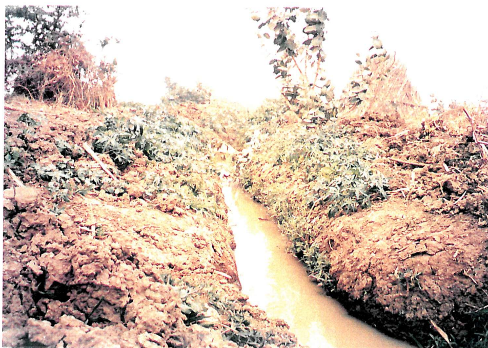
Plate10.7 Digging of main canal by farmers in order to enable water to flow further downstream
