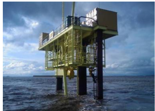
Figure 8-1: Pulse Stream 100 shallow flow prototype
