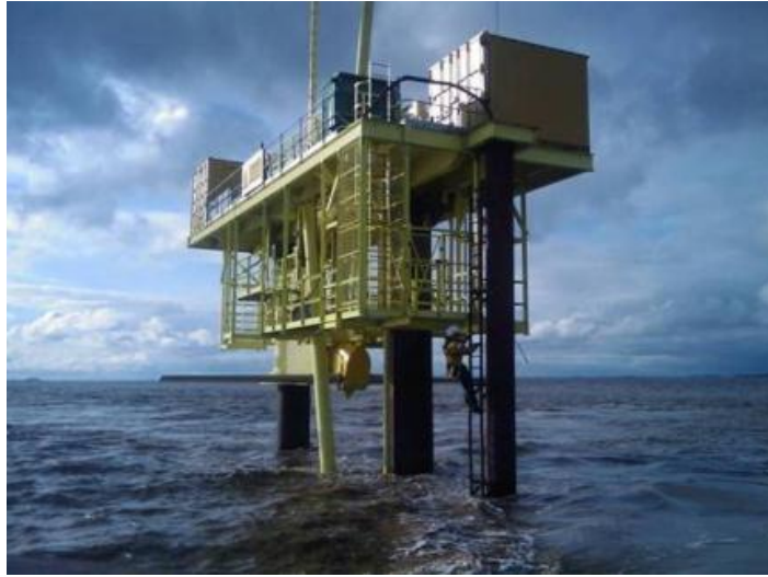
Figure 1-12: Pulse Stream 100 shallow flow prototype
