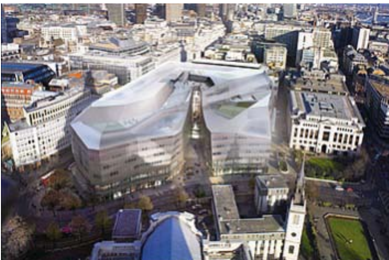
Figure 2. The One New Change Development, near St. Paul's Cathedral, has a Gross Floor Area of 52 000 m 2 made up of 31 000 m 2 of office space and 21 000 m 2 retail space.
