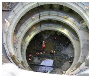
Figure 3. Energy Foundations Installed for the Crossrail Project in London.
