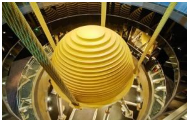
Figure 1.1 Dynamic vibration absorber is installed to the Taipei 101 to counteract vibrations in the building [8].
