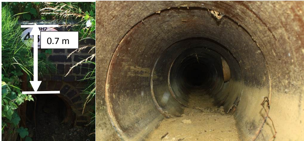
Figure 4: Culvert below the level crossing
