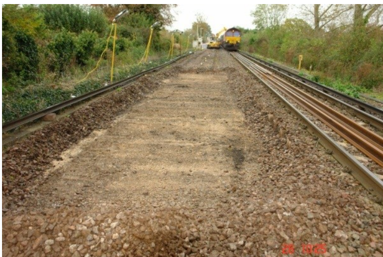
Figure 2: Formation being prepared for track renewal looking towards the nearby station from the level crossing
