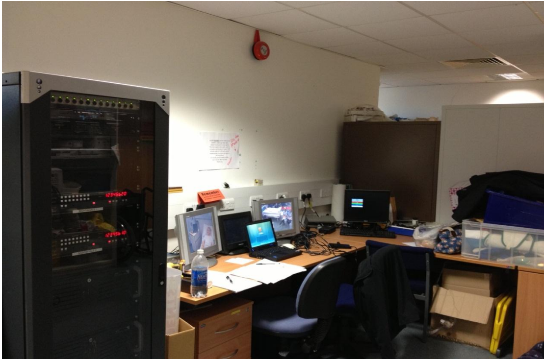
Figure 2: The control room.
