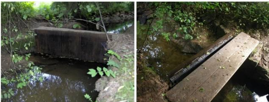
Figure 4.18: The Fish Screen. (left). Viewed from upstream, (right). Grill sections and support structure.
