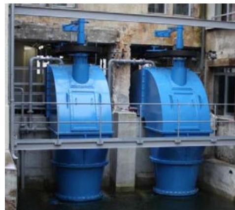
Figure 2.14: (top to bottom), Propellor devices (Applegate, 2010), Schematic of Siphonic Installation & 85 kW Siphon Turbines Installed at Vallorbe, (Choulot et. al. 2010).
