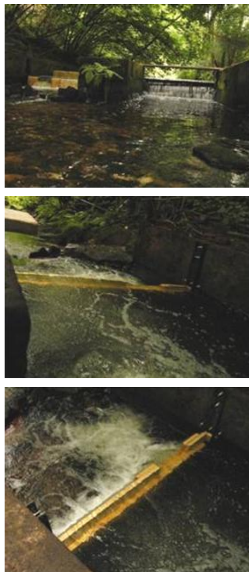
Figure 4.19: The Fish Pass. (left) from downstream, (centre) from upstream over one step, (right) one baffle.
