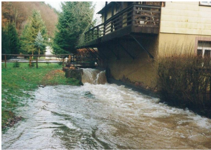
Figure 4.5: Flood Conditions at Partenstein Mill : Electrical Equipment needed to be mounted above the stone block seen here to the left of the water drop. (Kunkel Family Album)
