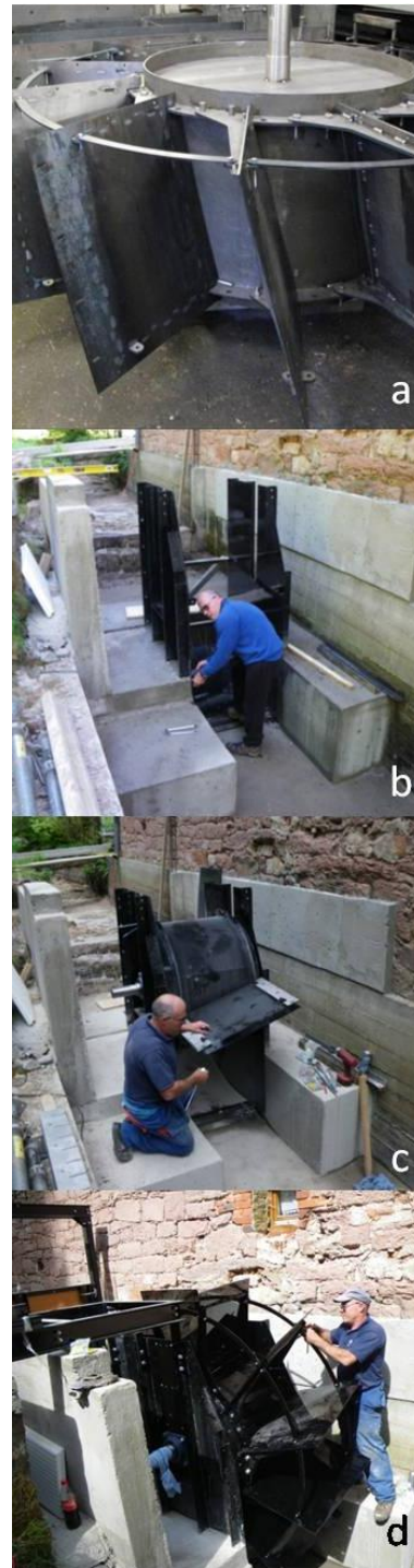
Figure 4.10: HPM Design a. Rotor during Fabrication, b. Side plates & panniers, c. Hub and Blade, d. Snub Ties
