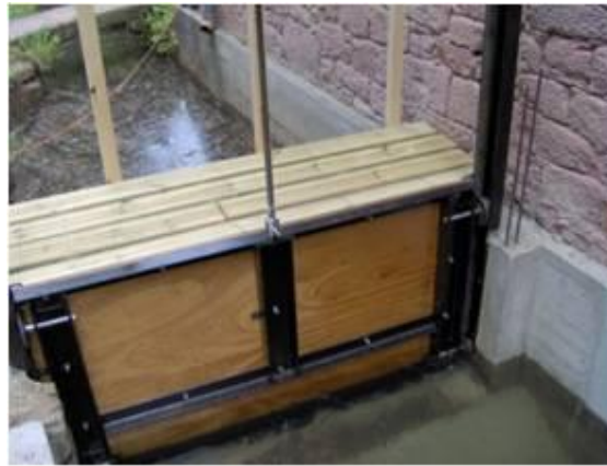
Figure 4.17: Sluice Gate, with marine ply blade, channel stiffeners and access platform.
