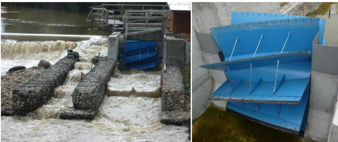
Figure 3.13: The HPM installation, River Iskar, Bulgaria. Operating in high water ( left ), Close up of welded steel rotor ( right ). (Bozhinova et.al. 2012)
