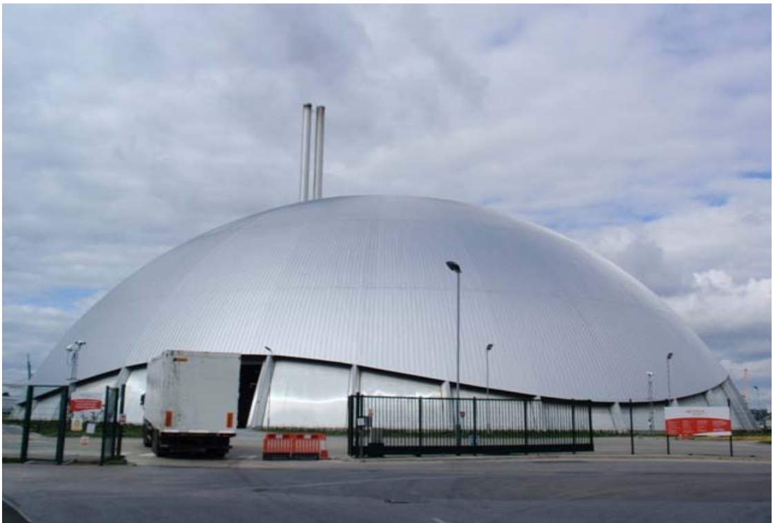
Figure 2.3 The Marchwood Energy Recovery Facility near Southampton, UK
