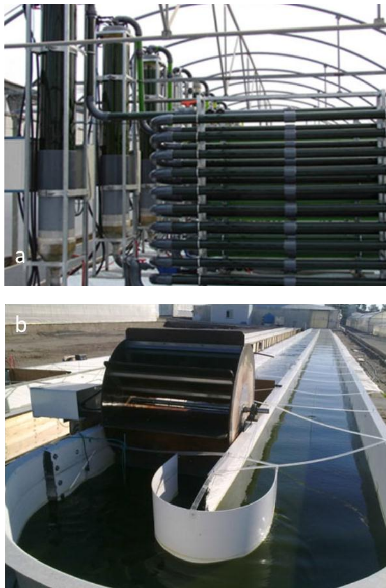
496 Figure 1. Algal cultivation facilities. (a) Tubular fence-type photobioreactor used to grow the 497 inoculum of Scenedesmus sp. (F.G. Acién Fernández et al., 2013) [40]. (b) Raceway reactor 498 in which the main algal culture was grown.
