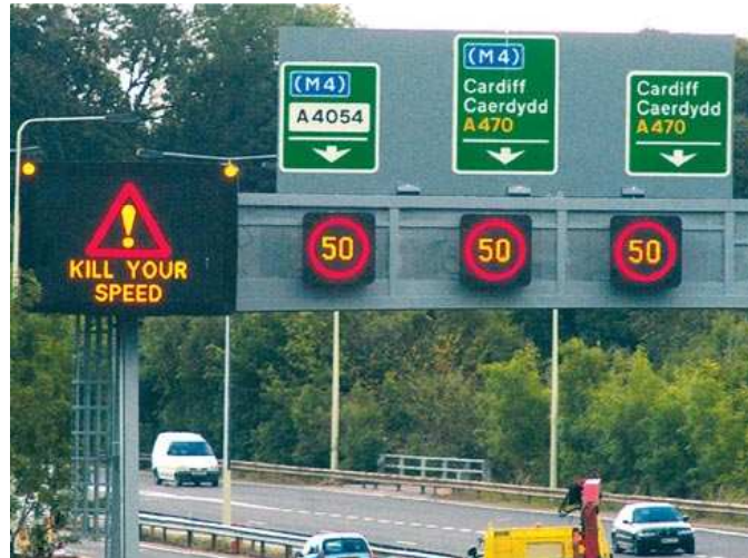
Figure 2-4 Photograph of Several Dynamic Message Signs (DMS) in the UK (Techspan 2013)
