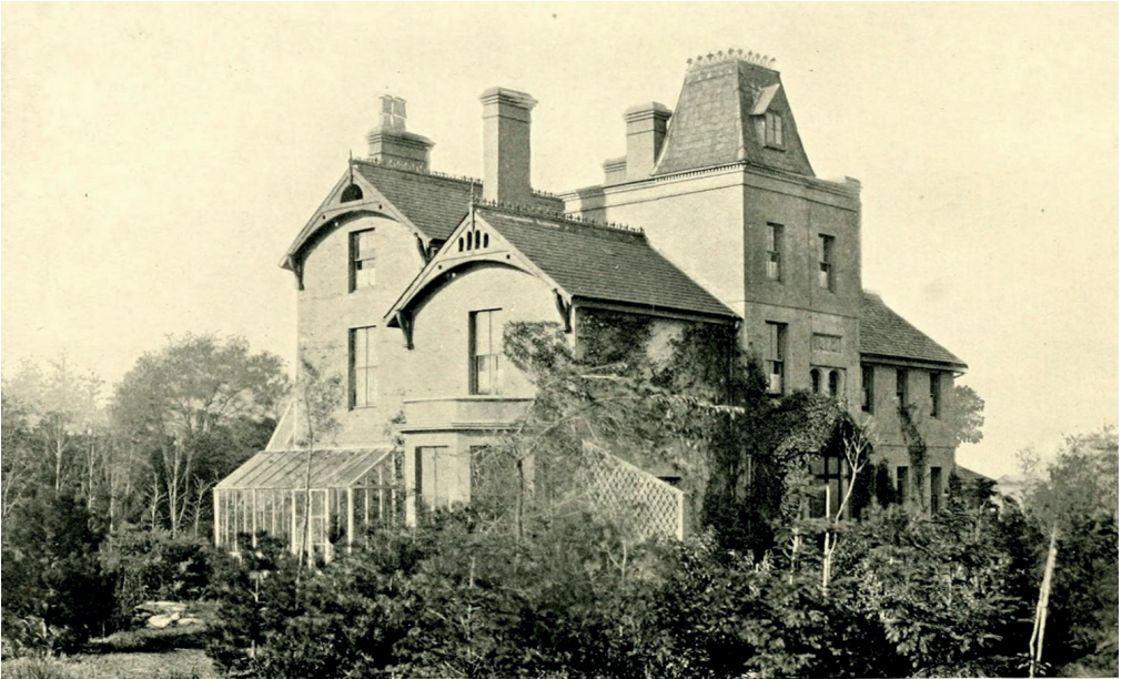
2.2 'The Dell', Grays, Essex. Wallace built this from shuttered concrete. Reproduced from Alfred Russel Wallace, My Life , 2 vols (London: Cassell & Company, 1905), vol 2, p 92 (facing).
