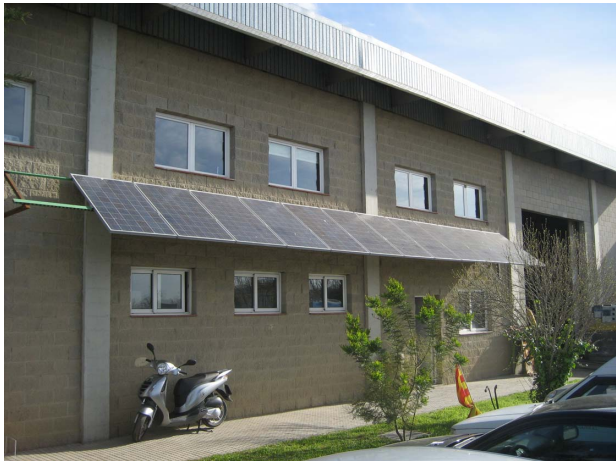
Figure 8. Stand-alone PV generator with 12 off-spec polycrystalline PV modules mounted on the façade of Sersall 95, S.L. in Castelló d'Empúries, Spain
