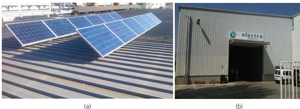
Figure 6. Grid-connected PV generator with 12 off-spec polycrystalline PV modules mounted on the roof of Electra Caldense in Caldes de Montbui, Spain (Arranz et al. , 2013b)
