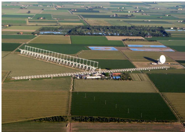
Figure 1: A top view of the Medicina Radioastronomical Station. In the foreground the Northern Cross T-shaped array.
