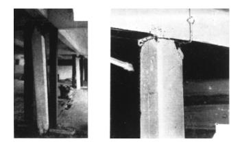
Figure 2. Shear failures due to blast (Baker et al., 1948)
