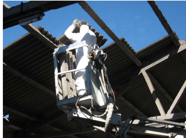
Figure 5. Careful removal of asbestos in site 3
