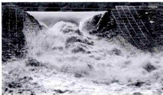
Fig.1 The instant of dam break
