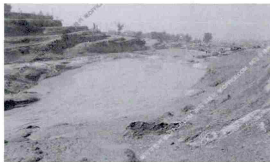
Fig.2 Dam accident in Xiangfen (Xi'an, 1980)
