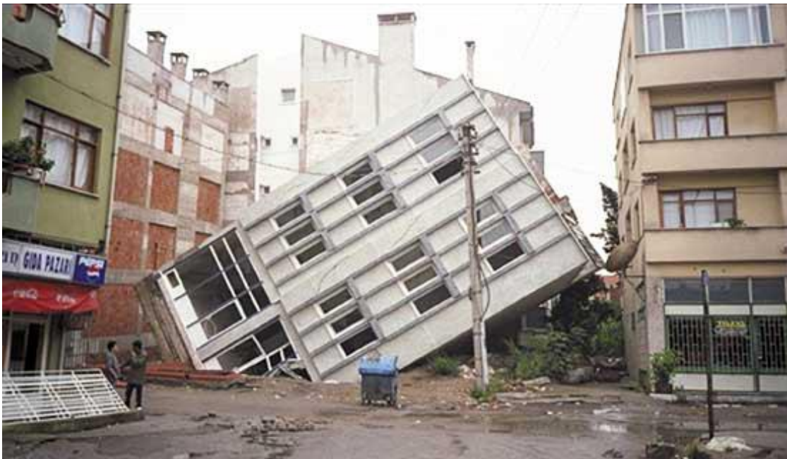
Figure 1.13: Example of the effects of soil liquefaction on a large scale, as occurs during earthquakes. (Image from http://7bcore2.wikispaces.com/Glossary accessed 18/10/2013).
