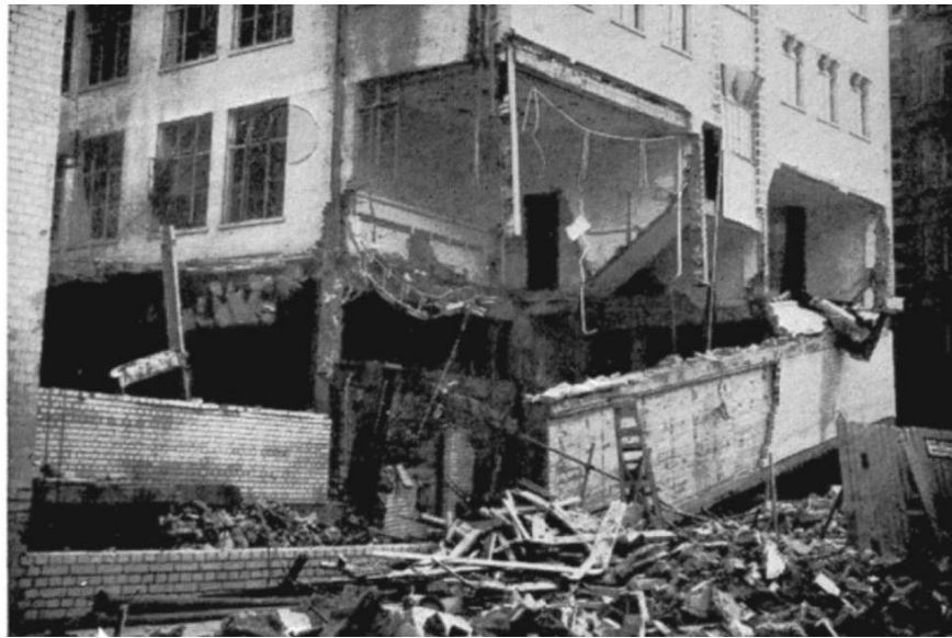
Figure 2.1: Front wall unsupported due to the unseating of a girder, Byfield (2006)
