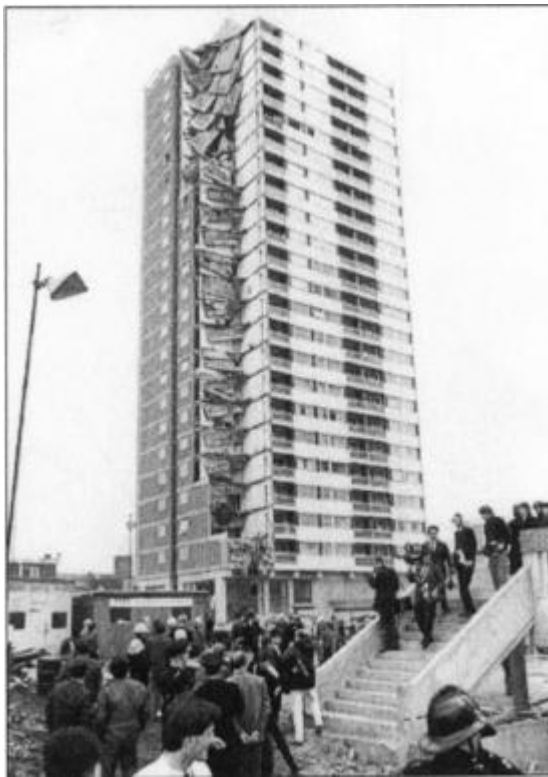
Figure 2.2: Progressive collapse at Ronan Point, Pearson and Delatte (2005).
