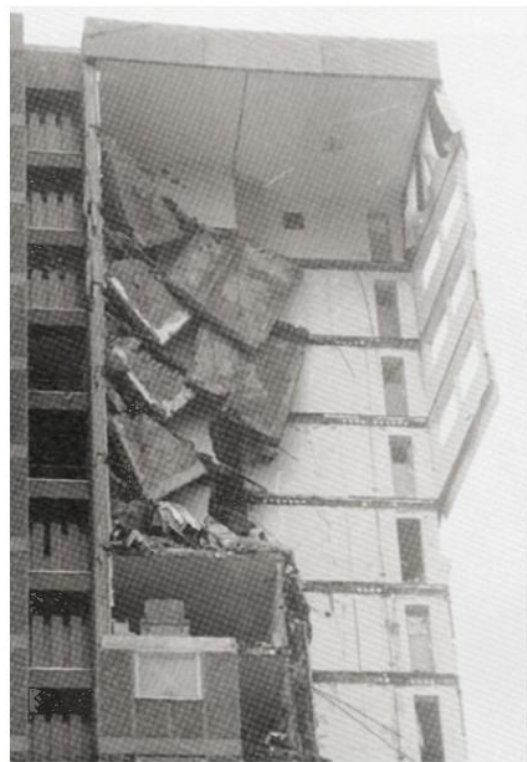
Figure 2.3: Close up of the damage at Ronan Point, Bussell and Jones (2010).
