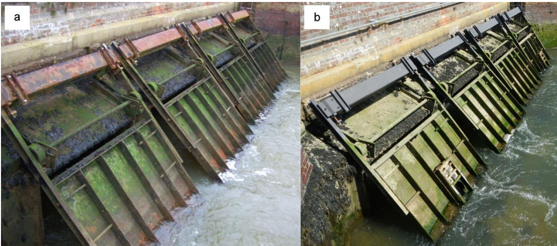
Fig. 7.2. (a) Four counterbalanced top-hung tide gates on the River Meon at Hill Head, Hampshire, UK, in 2011 (year 1), pre installation of orifices; (b) orifices were installed in two of the gates in 2012 (year 2).
