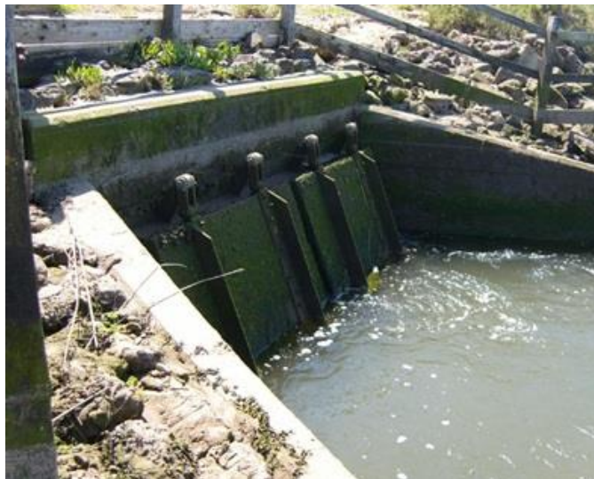
Fig. 5.3. Tide Gate 2 in the River Stiffkey, North Norfolk, UK, consisting of two top-hung un-counterbalanced gates.
