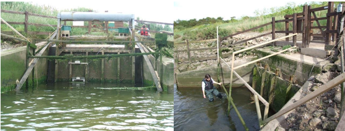
Fig. 4.1. HDX PIT loops (PLs) located immediately downstream of Tide Gates 1 (left) and 2 (right) in the River Stiffkey, UK.
