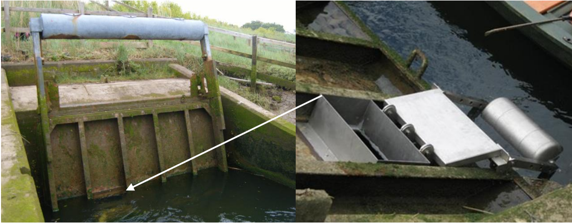
Fig. 5.2. Left: Tide Gate 1 in the River Stiffkey, North Norfolk, UK, a counterbalanced top-hung gate. Right: An orifice fish pass installed in Gate 1.
