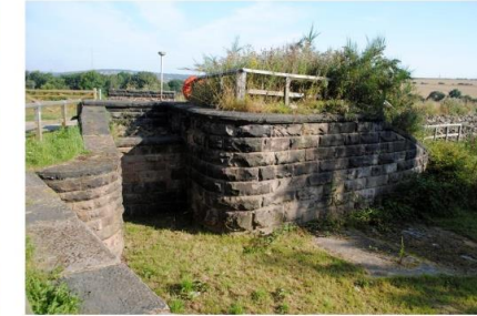
6. Pre 2007 (1943) storm overflow at Ulley reservoir
