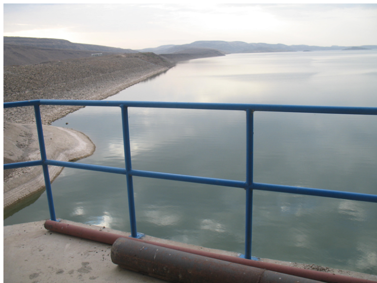
Fig. 2. Reservoir view seen from the intake tower.
