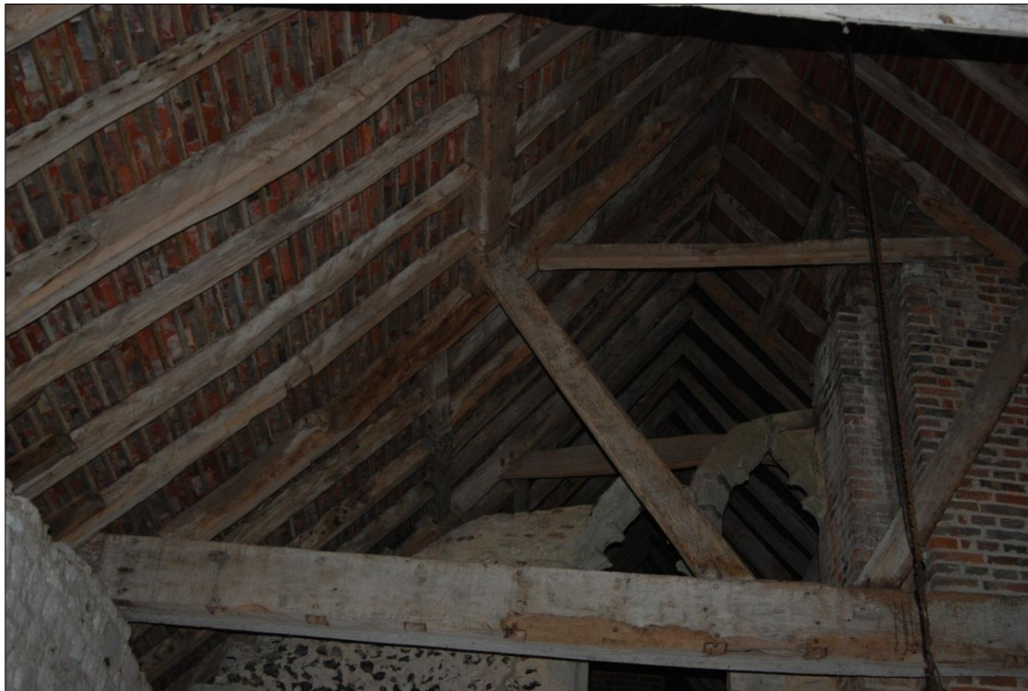
Figure 88: Wilmington Priory Roof without crown post
