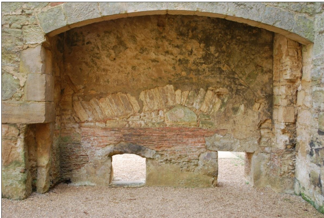
Figure 56: Western range fireplace. Here the opening of the fireplace has changed direction multiple times.
