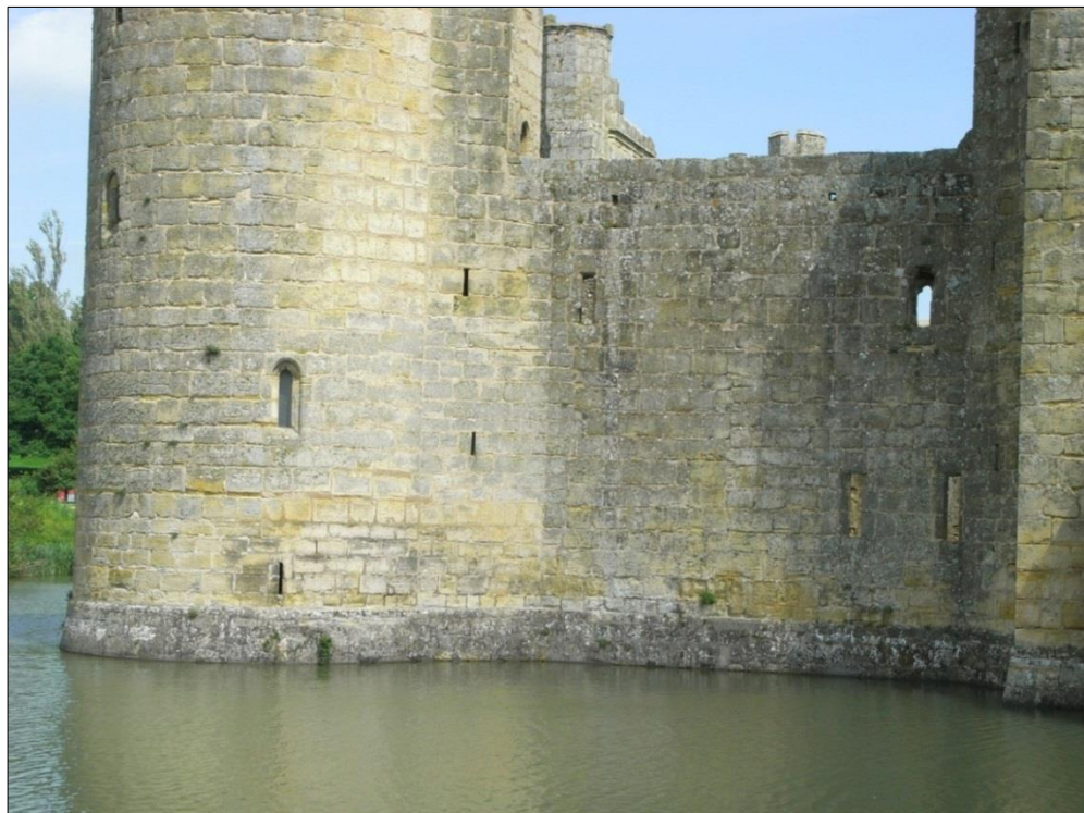
Figure 54: Straight Joint in masonry on the northern elevation. This probably represents the break between two seasons of building works during construction.
