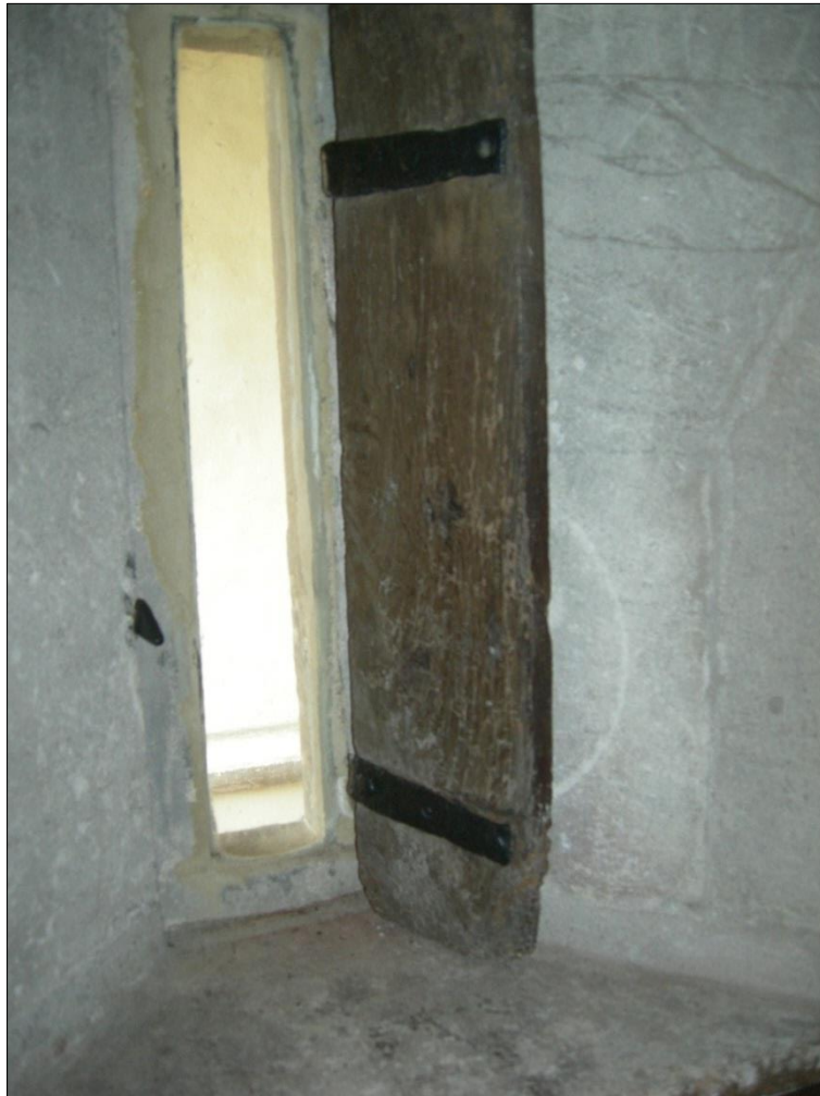
Figure 105: Hinges and latches from an original shutter at Great Chalfield, Wiltshire.
