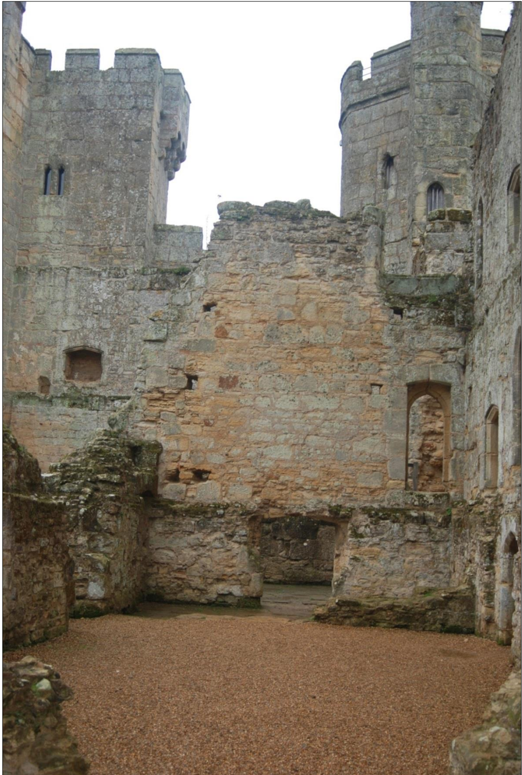
Figure 103: Wall at the northern end of the eastern range. The doorway shows which way the door would have pulled open based on the indentation in the stonework.
