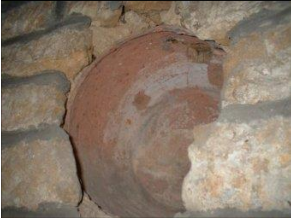
Figure 35: Close-up of the acoustical jars at St Andrew's Church in Lyddington (Murphy 2004)
