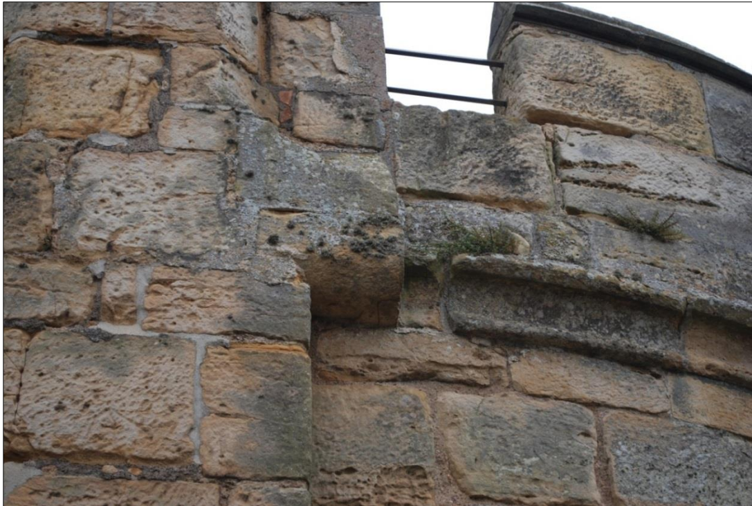
Figure 55: Corbel and string course on the north-western tower. This is one of the pieces of evidence for a change of mind during the construction of the castle.
