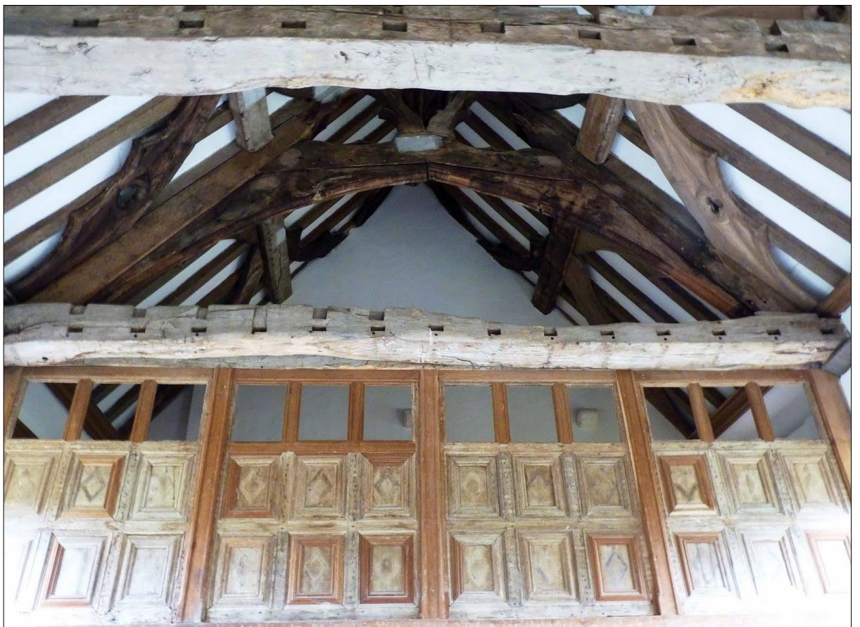
Figure 82: Plank and muntin screen at Fiddleford Manor, Dorset (Tiller 2012)
