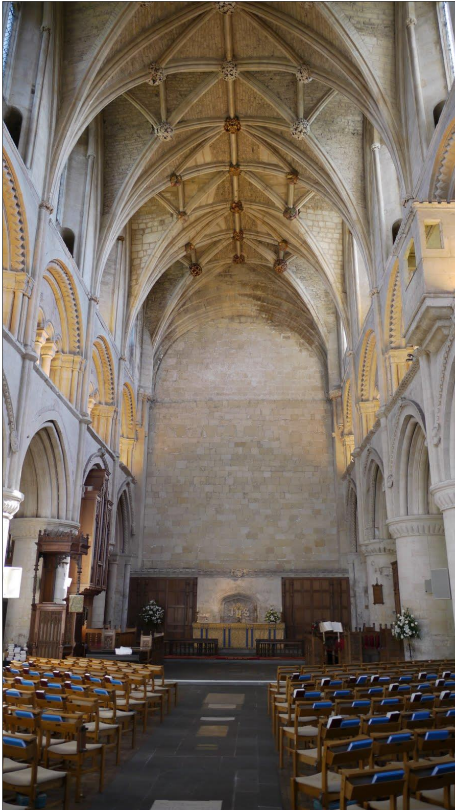
Figure 13: Malmesbury Abbey, Wiltshire. This building shows how the presence of aisles in a hall breaks up the width of the room. Unlike in secular buildings the use of aisles continued after the development of the hammer beam roof; in buildings with both stone and wood roofs.
