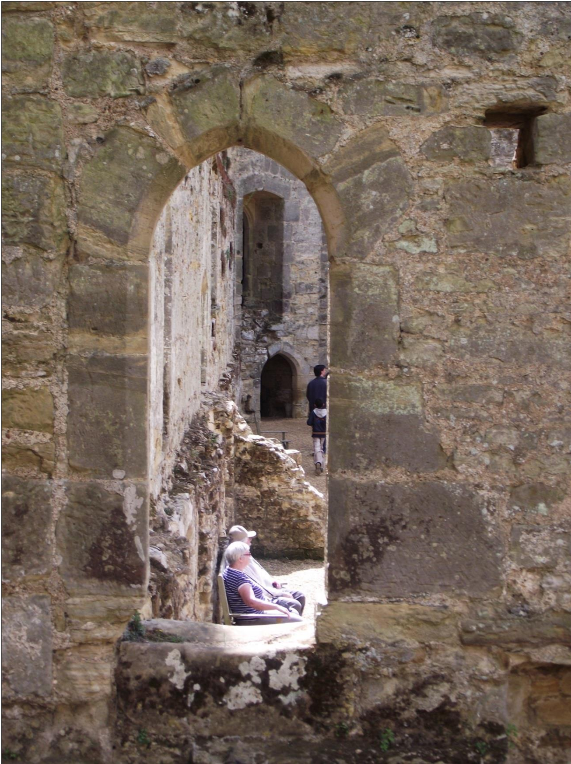
Figure 84: The eastern elevation at Bodiam looking south. Here a ridge can be seen running along the wall edge (above the people sitting on the bench) this is the ridge the floor would have rested on.
