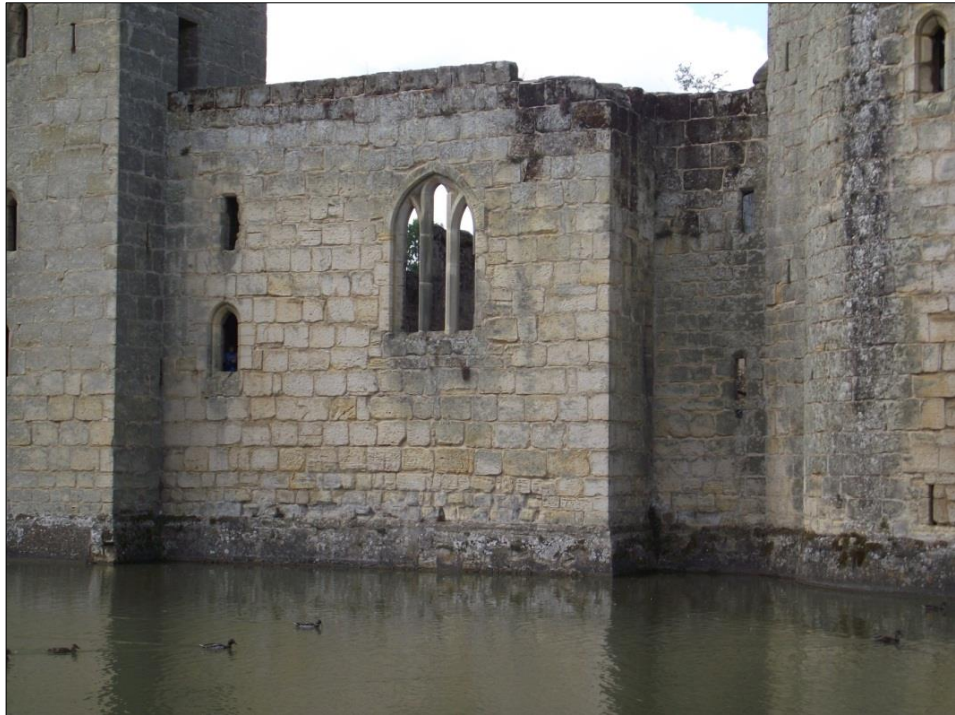
Figure 45: Eastern elevation showing the misaligned Chapel wall, photo taken from the east. This is one of the examples of how the building is not as symmetrical as it first appears.
