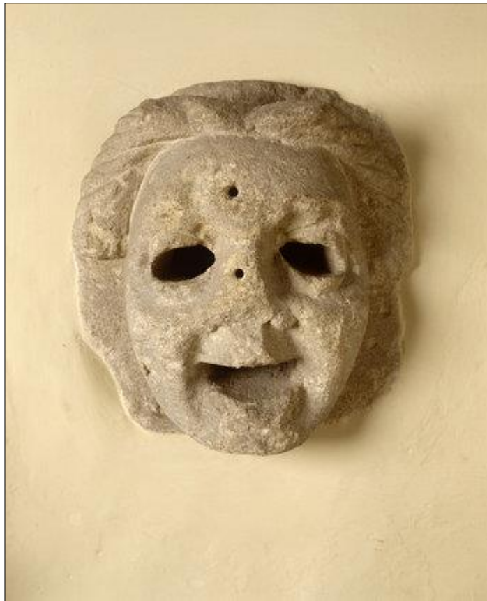
Figure 20: A stone mask squint at Great Chalfield. This is found in the upper walls of the great hall; this allows the hall to be overlooked from the withdrawing chambers ©NTPL/Nadia Mackenzie (Mackenzie 2014a).
