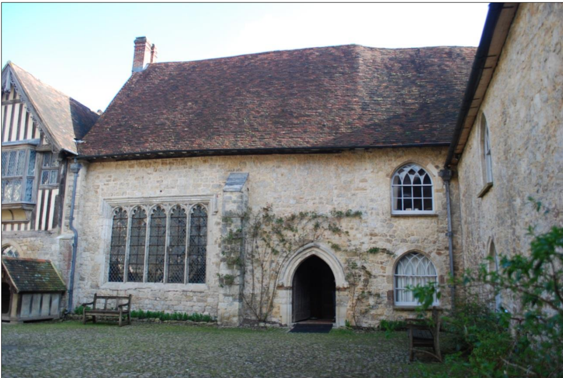
Figure 247: Insertion of the perpendicular window in to the Great Hall. We can also see the lack of porch. The change in roof line shows the removal of the services as does a straight joint in the masonry directly below.
