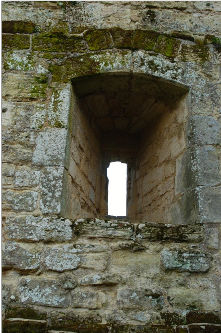
Figure 182: Window on the eastern elevation. You can see clearly two hollows to the right of the image where fixtures held the window shutter in place.
