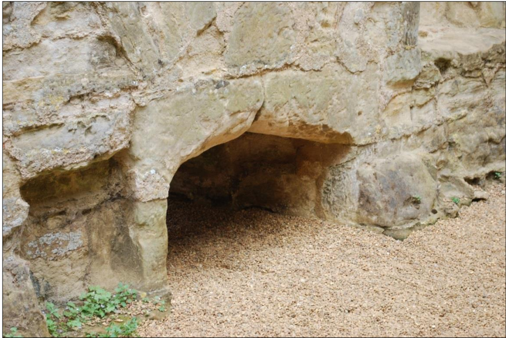
Figure 53: Kitchen window below floor level. Probably evidence for a cellar for storage below the buttery.
