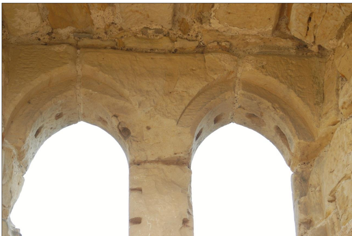
Figure 102: View of the window seats in the private apartments. This photo shows how the bars have been forced out of the windows and the positions of the bars.
