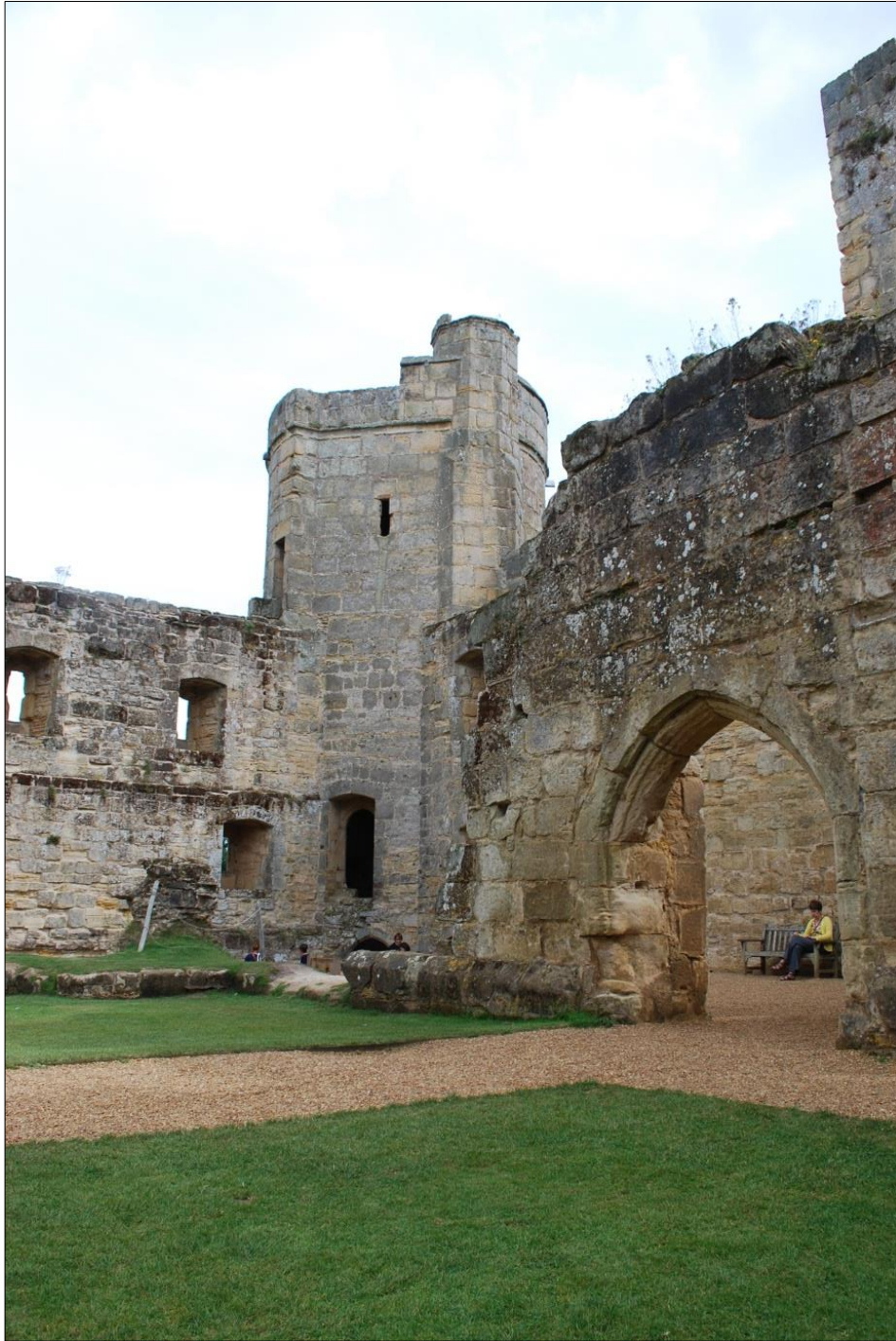
Figure 47: South-east tower taken from the west of the courtyard. Compared to Figure 46 the internal appearance of the tower is different. It “chamfers” the internal curve.
