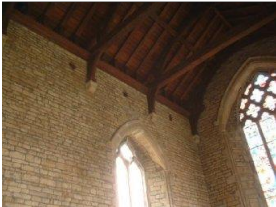
Figure 34: Acoustical jars in situ at St Andrew's church in Lyddington (Murphy 2004). The concept of the jars was designed by Vitruvius to make sound
