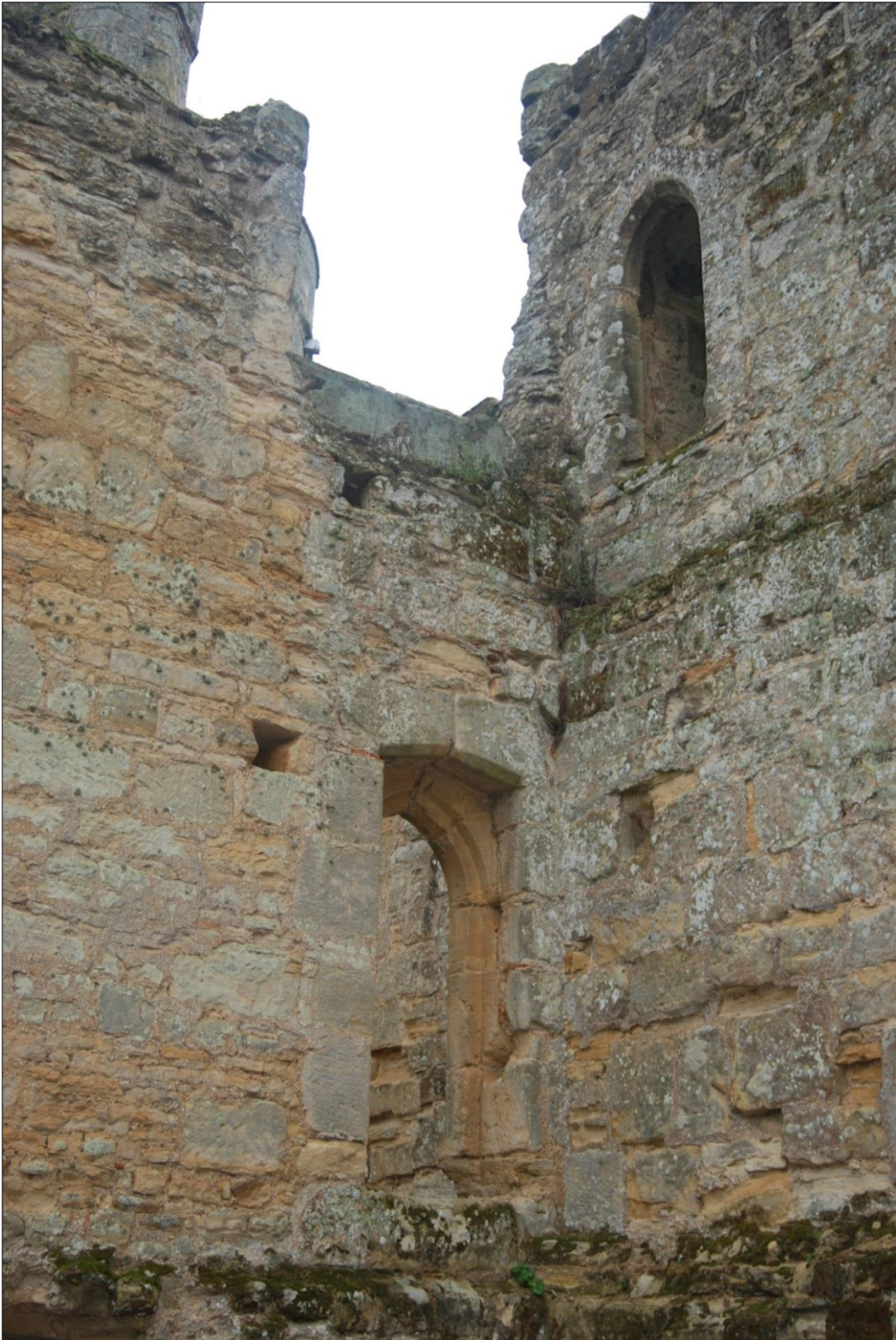
Figure 104: Northern doorway in more detail (closer view of Figure 103), note detail on recess which shows where the door would have been placed.
