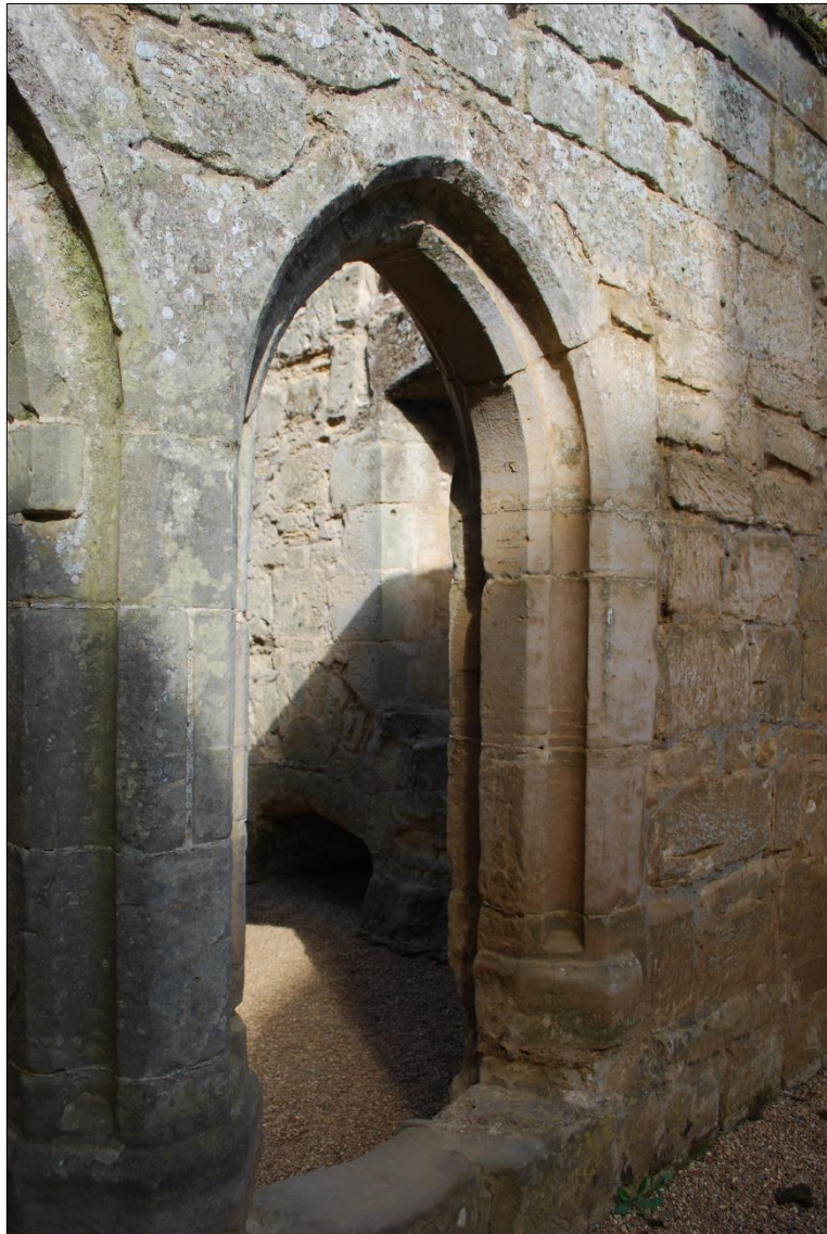
Figure 256: Window at Bodiam Castle, note the chamfered edges of the window. These are where a right angled corner has been cut off to create a smooth edge.
