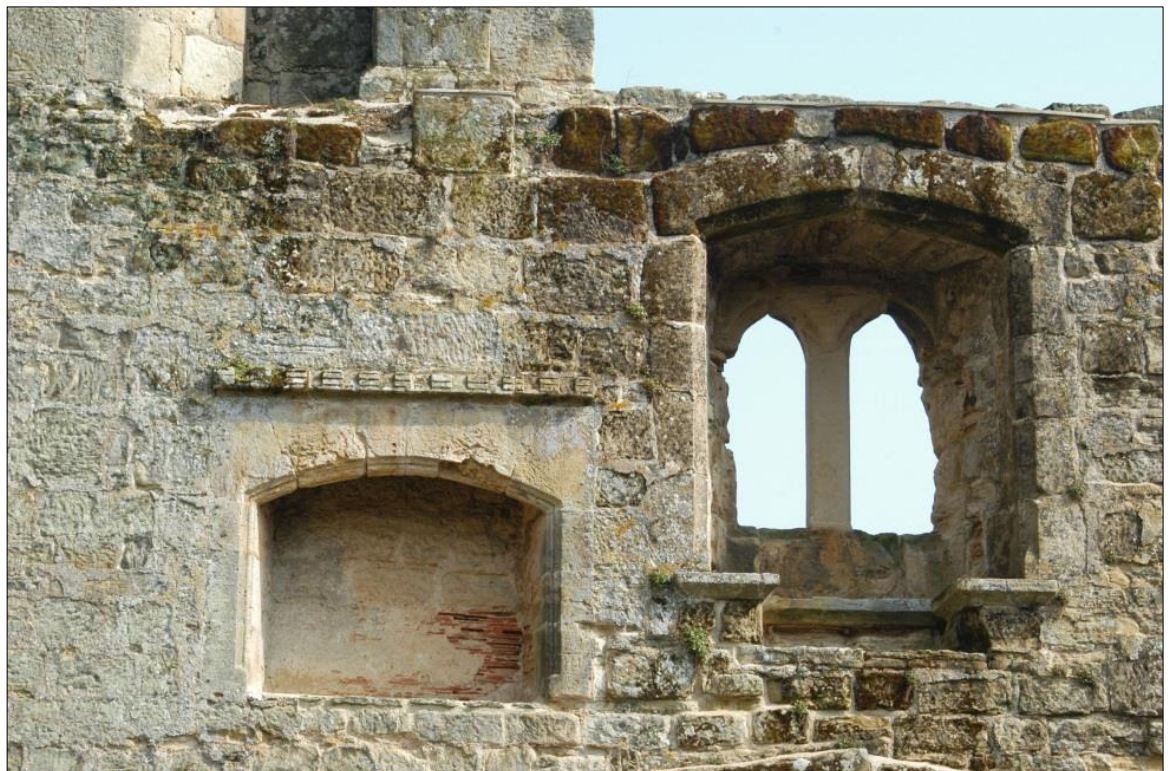
Figure 181: Window seat built into the eastern elevation in the upper apartment. Photo taken from the west looking east, there is no evidence in the brick work for the removal of shutters.
