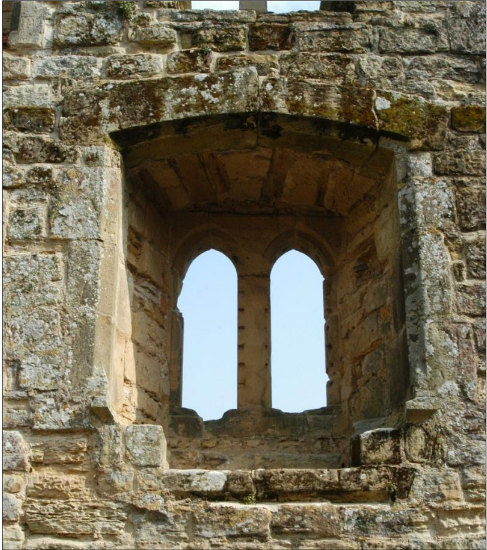
Figure 164: One view of the window seat in the eastern elevation. The position of the window bars can clearly be seen in the masonry
