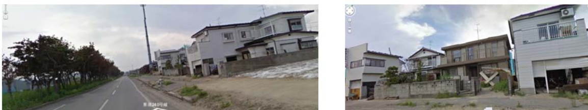
Figure 11 Buildings in Area B behind the port in Ishinomaki showing evidence of sheltering by trees (GSV, 2013c)
